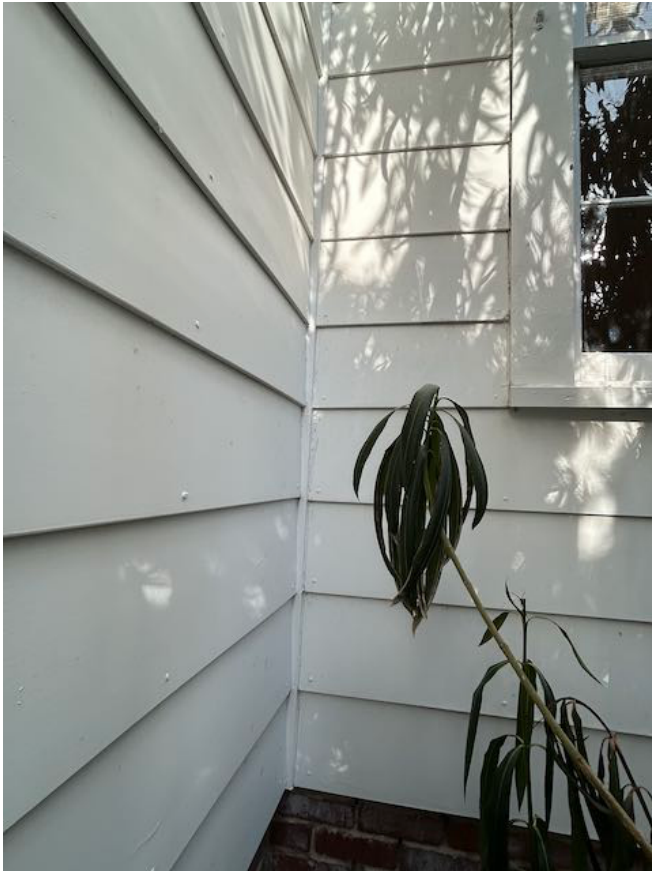
PHOTO 7: Detail of how the lapped, manufactured siding of the bump-out aligns with the wood German-profile siding of the historic home. This relationship will be preserved.
