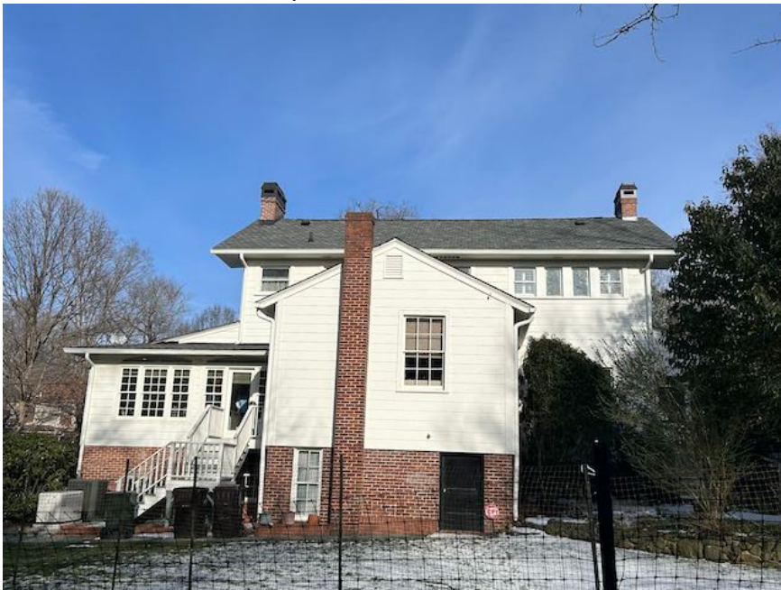
PHOTO 4: West (rear) elevation. The bump-out can be seen here, and this face will be obscured by the proposed addition, which would require demolition of the chimney. The (2) double-hung one-over-one upper windows on the south (righthand) side are proposed to be replaced.
