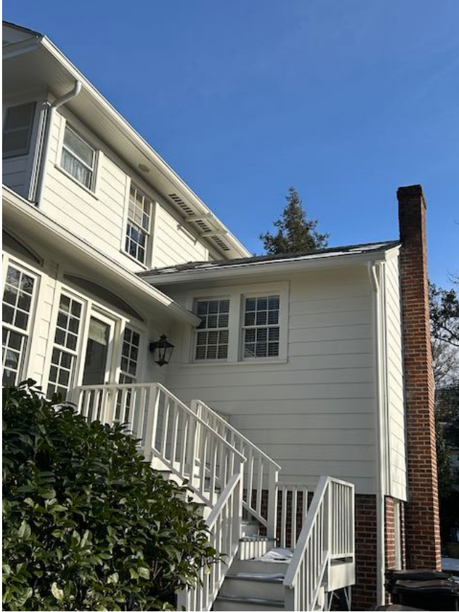
PHOTO 5: North elevation of bump-out. Note the conflict between the kitchen roof and the double-window of the bump-out. The upper six-over-six double-hung is proposed to be replaced.
