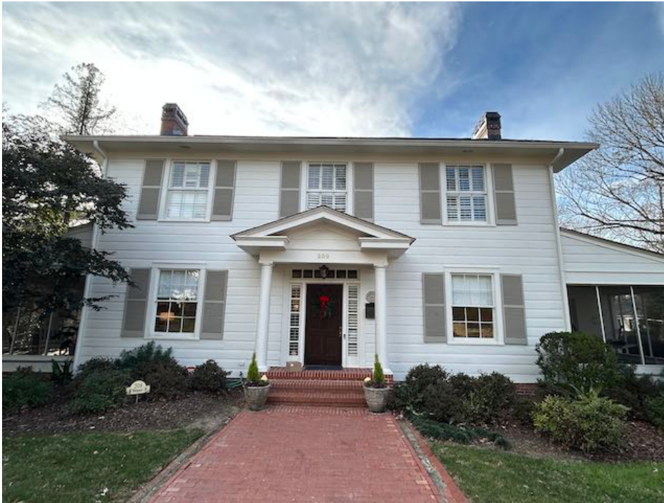
PHOTO 1: Primary façade (east). All five 6-over-6 double-hung windows seen here are proposed to be replaced.
