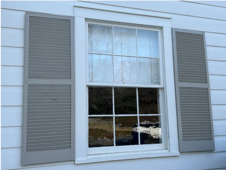
PHOTO 8: Detail of six-over-six double-hung that is proposed to be replaced.
