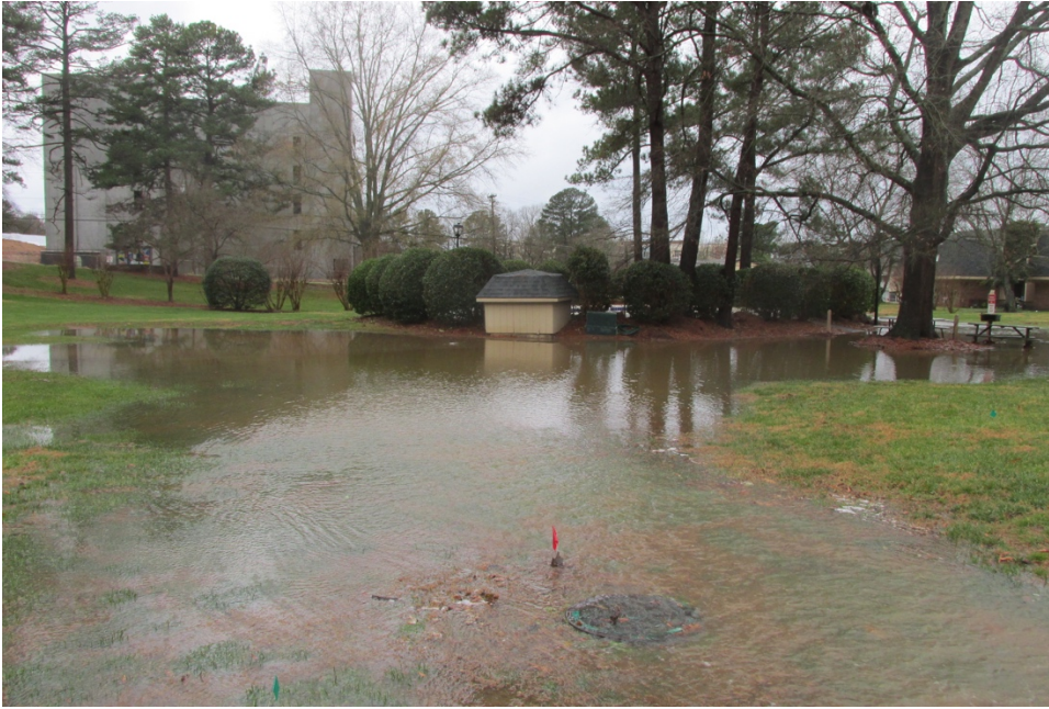
Photo 4: Flooding from the pool area past the 100 Building to the collection drain under Ephesus Church Road.
