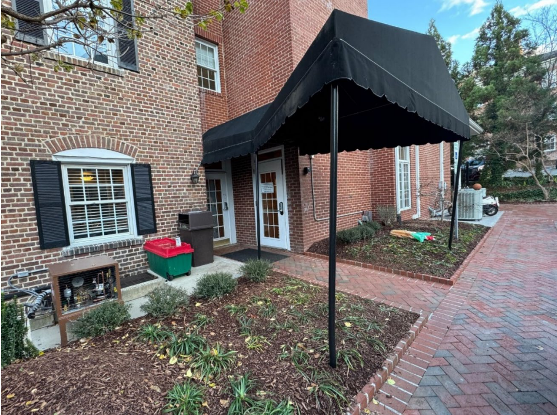
Existing rear entrance canopy
