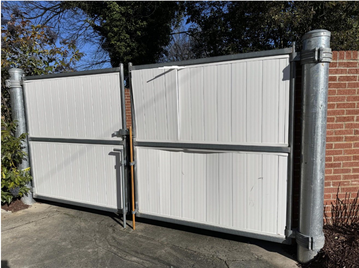
Existing dumpster gates
