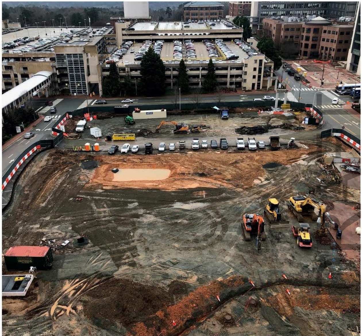
SITWORK PROGRESS VIEW TO THE SOUTH
