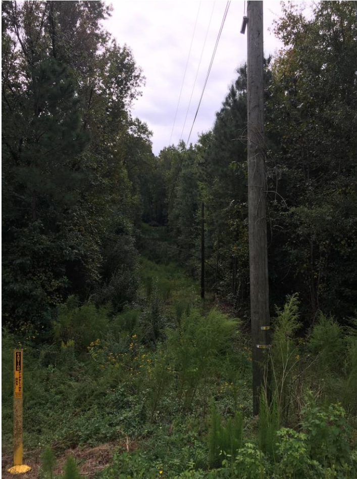
View Into Site At Electric Corridor
