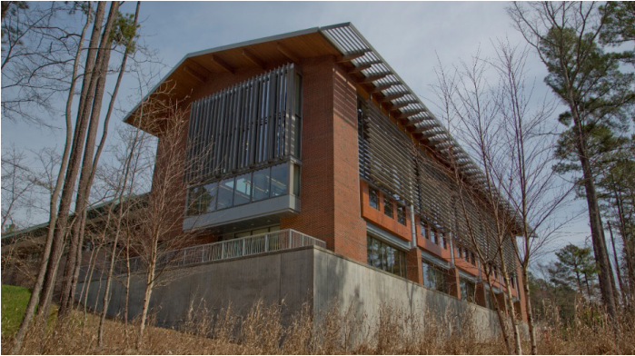
The 2013 expansion of the Chapel Hill Public Library achieved a LEED Silver rating from the U.S. Green Building Council.
