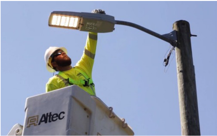
Duke Energy contractor testing a newly installed LED streetlight
