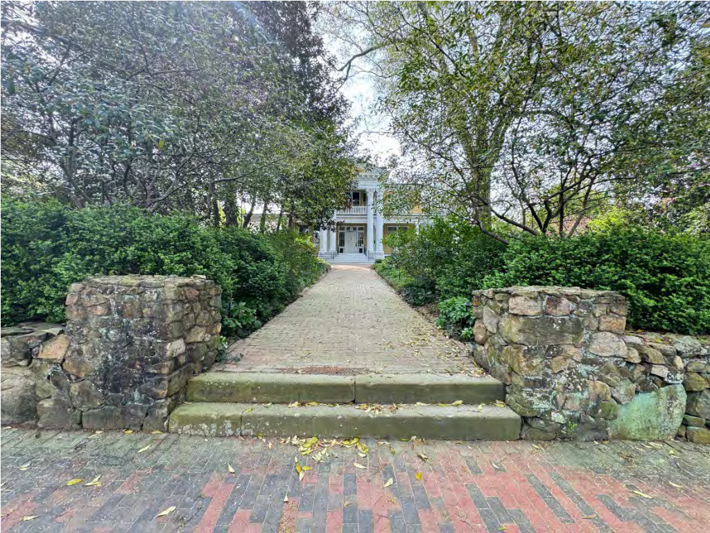
VIEW FROM E. FRANKLIN STREET SIDEWALK
