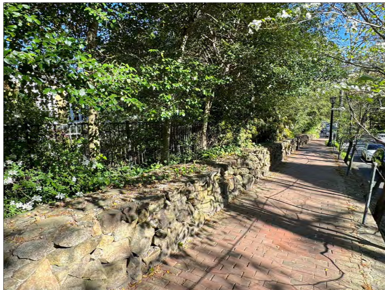
EXISTING CONDITIONS SHOWING EXISTING ALUMINUM 4 FT HEIGHT FENCE along SIDEWALK at RALEIGH ROAD
