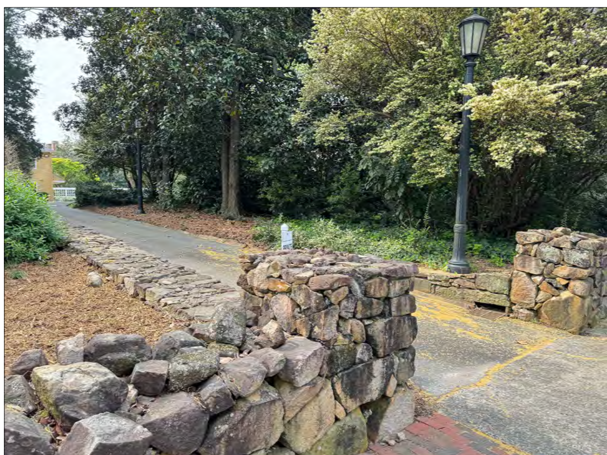
3. View of Driveway from sidewalk along E. Franklin St. showing stone piers
