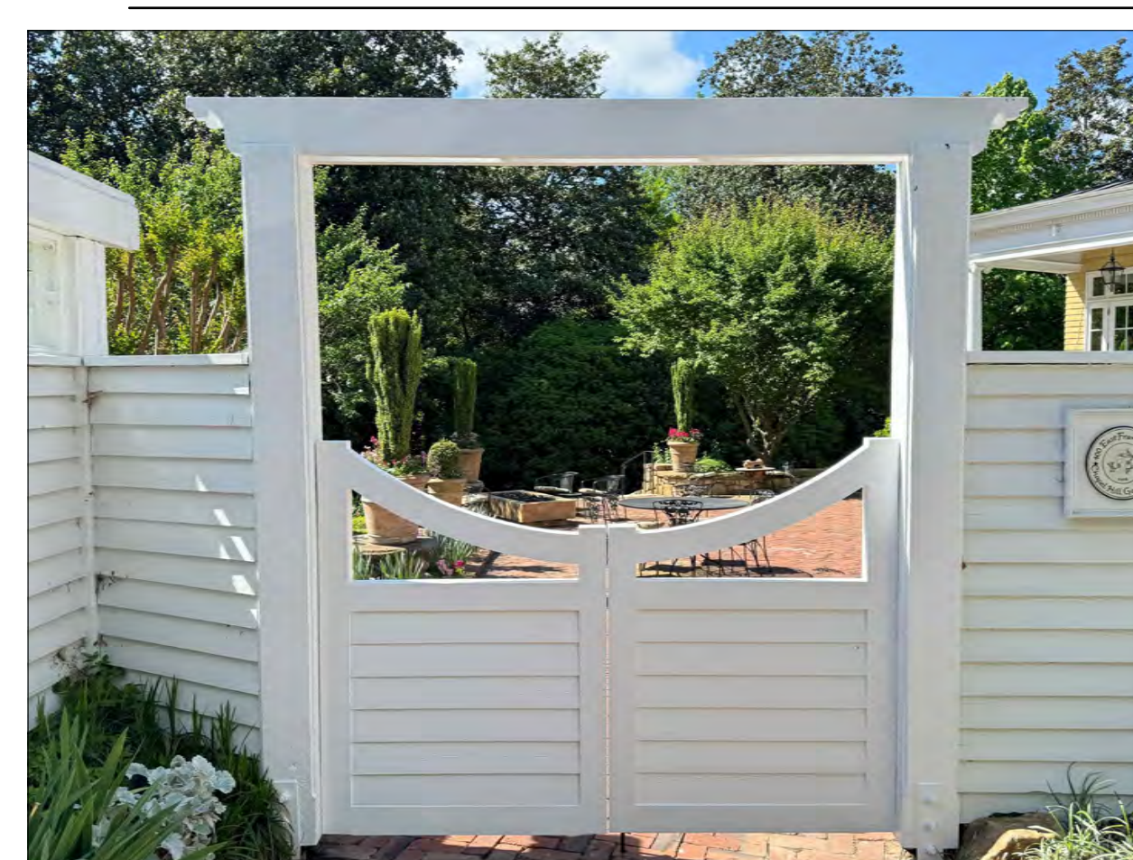
UNC President's Residence Garden Gate (with swooping gate detail - Front Elevation view)
