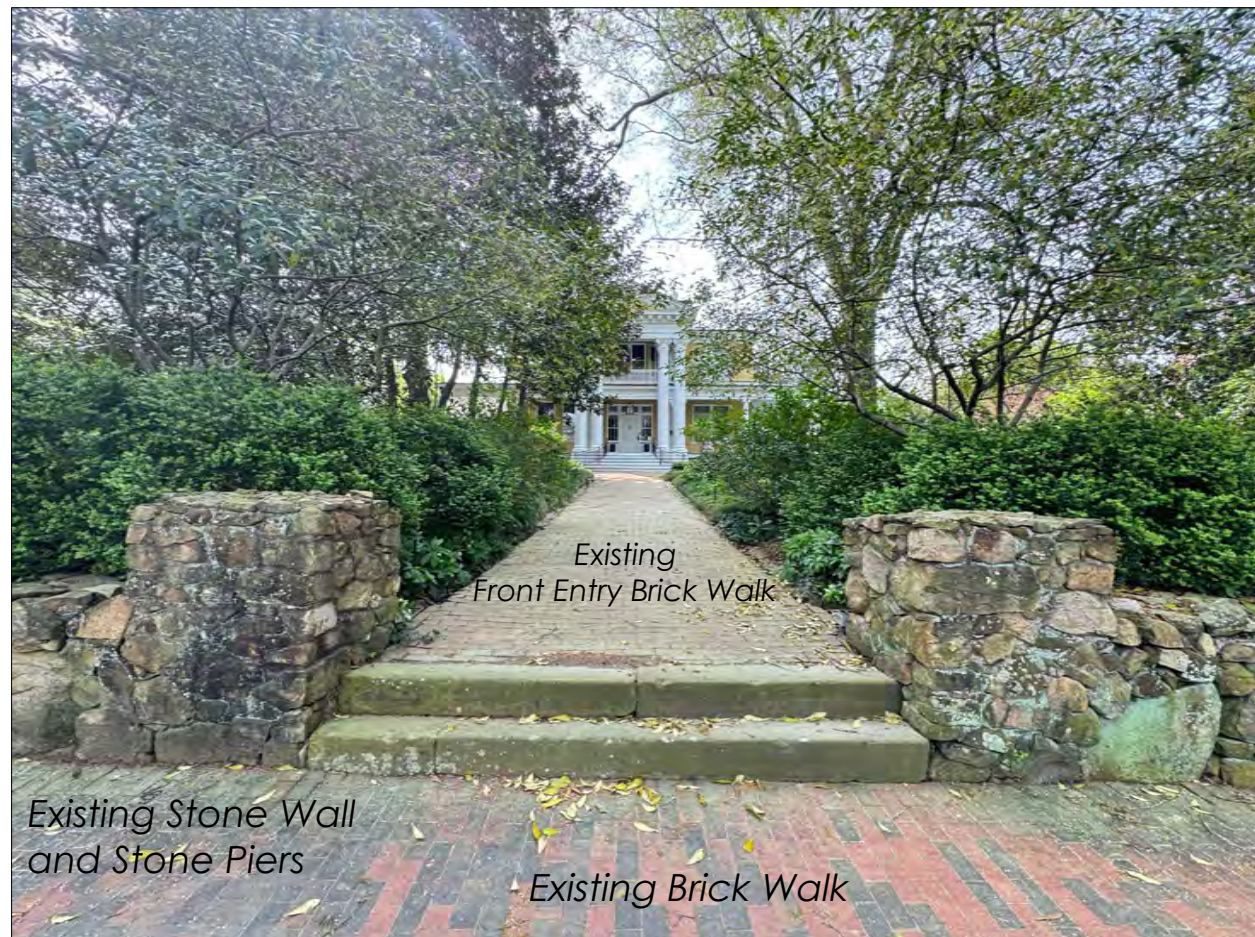
EXISTING CONDITIONS VIEW along SIDEWALK at 400 E. FRANKLIN ST.
