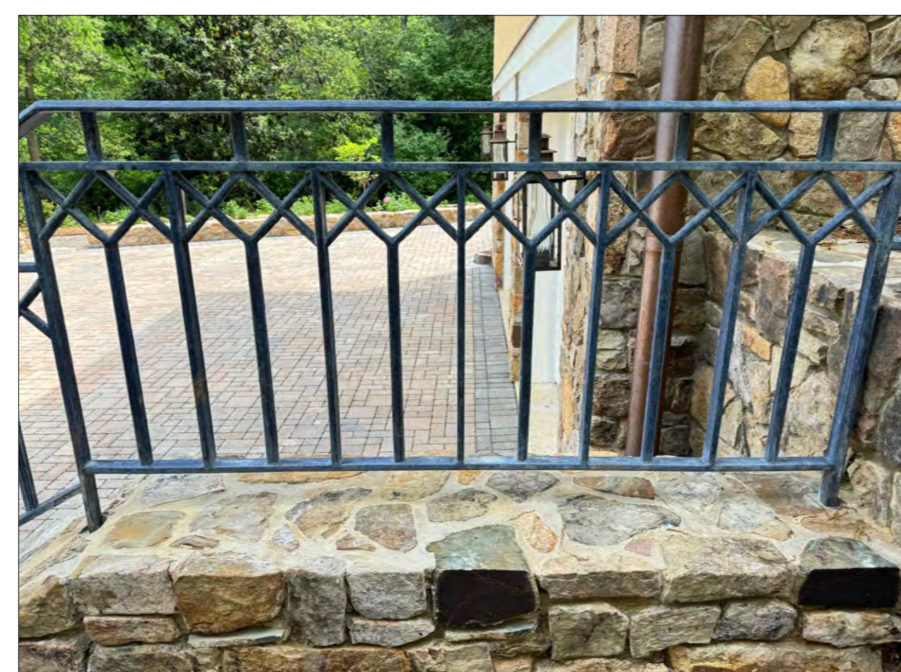
EXAMPLE DETAIL for BARRIER RAIL at Front Entry Walk
