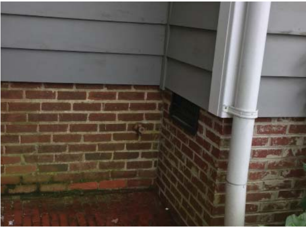
Existing condition, northeast corner
