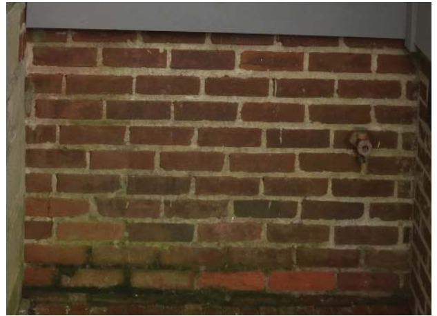
Existing running brick bond
