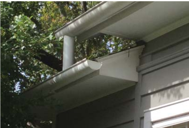
Existing eave & soffit
