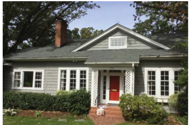
Existing windows in wall with horizontal siding.
