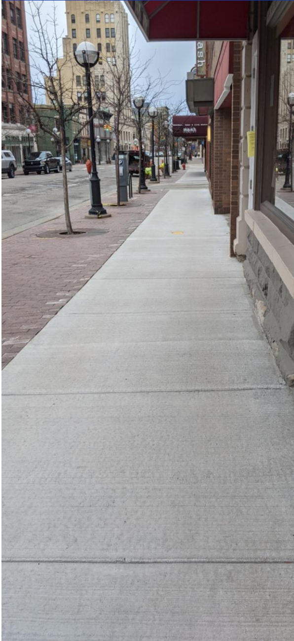
Sidewalk and Paver Repair
