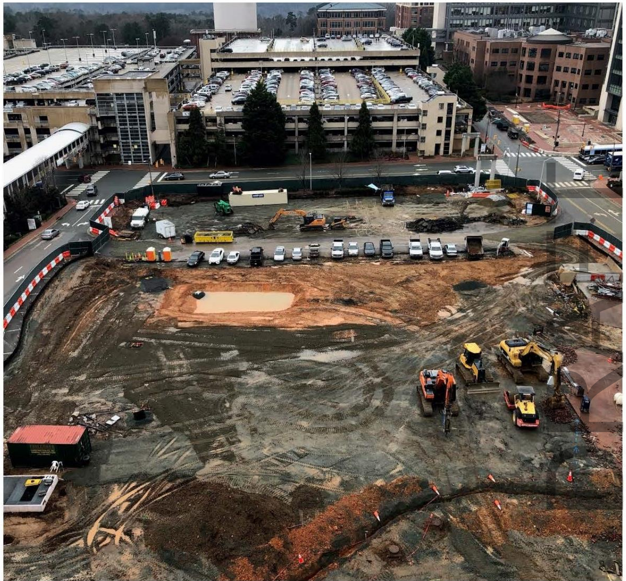
SITWORK PROGRESS VIEW TO THE SOUTH
