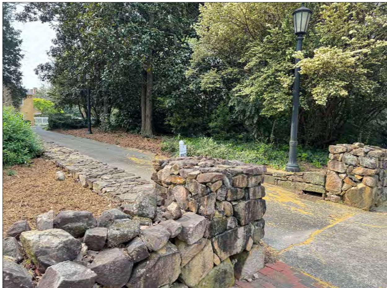
3. View of Driveway from sidewalk along E. Franklin St. showing stone piers
