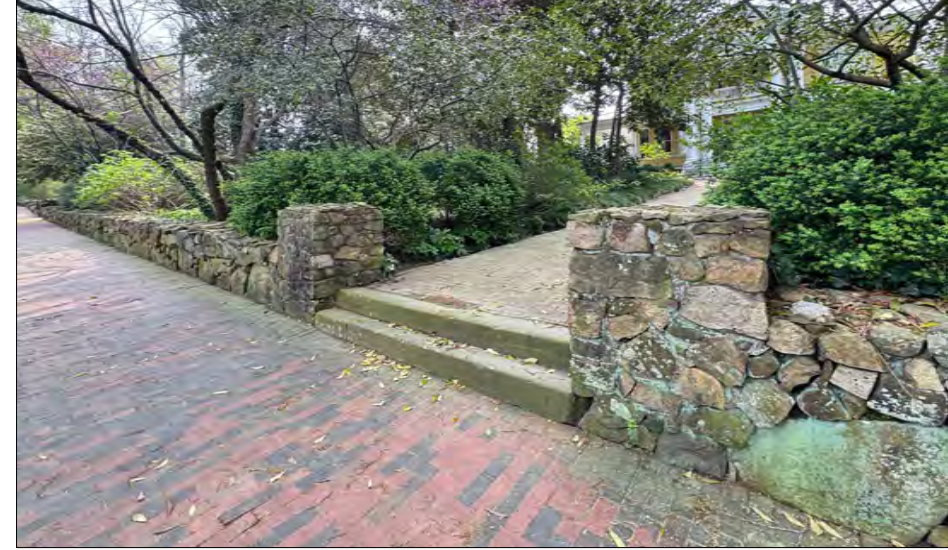
EXISTING CONDITIONS VIEW along SIDEWALK at 400 E. FRANKLIN ST.
