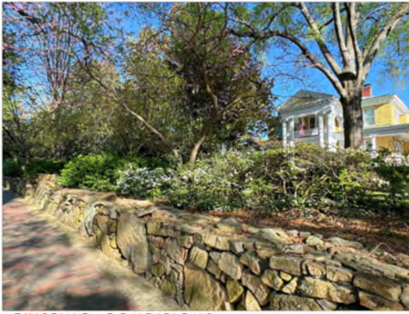
EXISTING CONDITIONS VIEW along SIDEWALK at 400 E. FRANKLIN ST.
