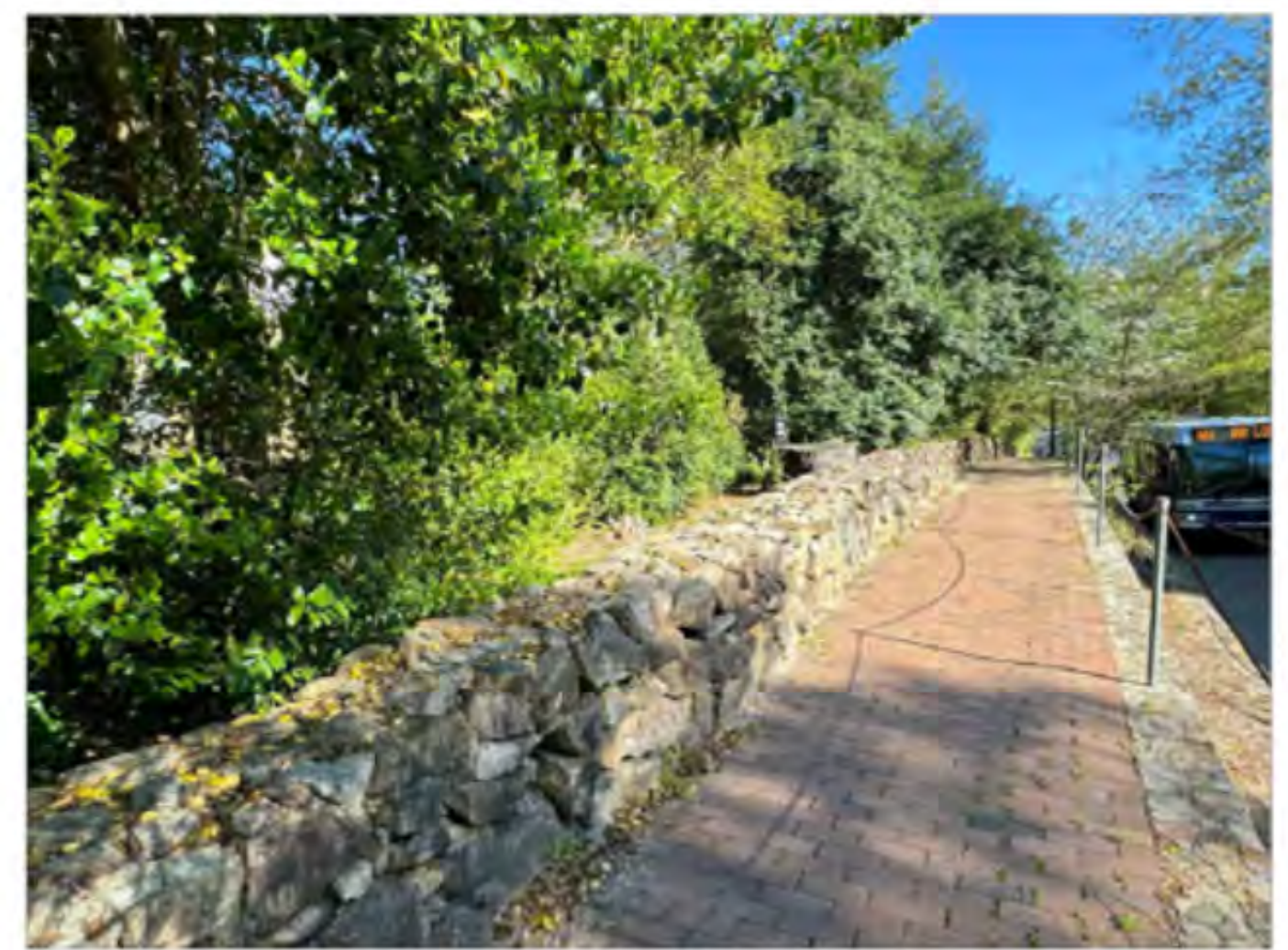
EXISTING CONDITIONS VIEW along SIDEWALK at RALEIGH ROAD
