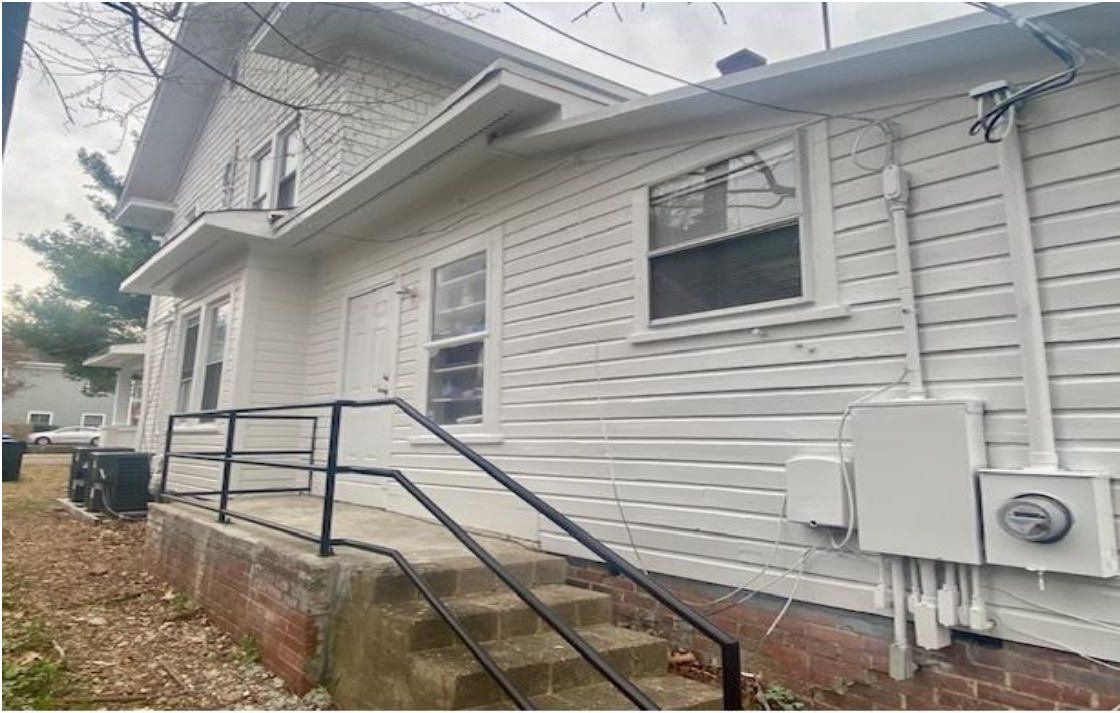
View of east side from rear of property
