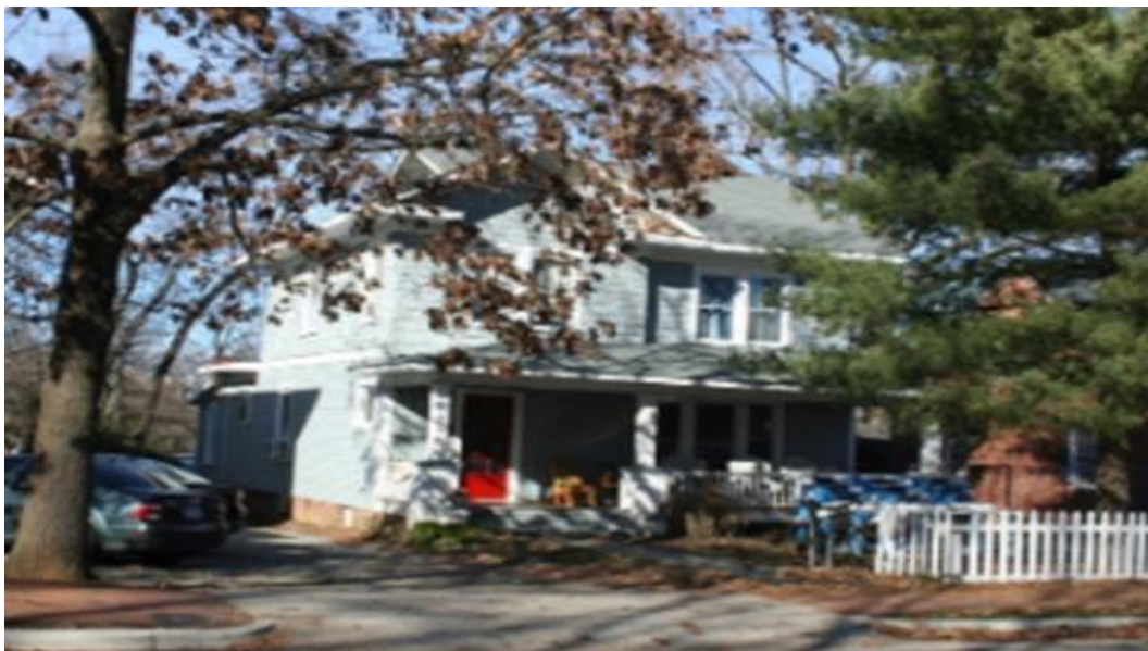
Older photo of subject property found at www.historicchapelhill.org
