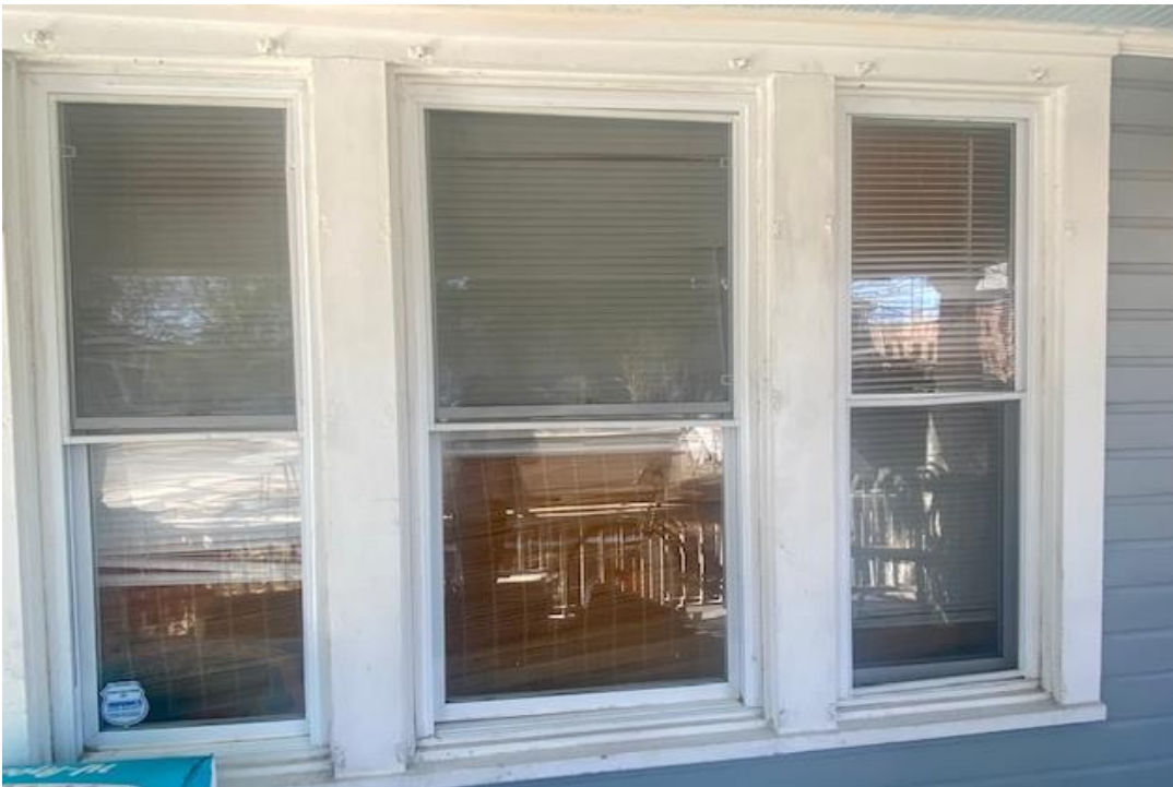
Closer view of existing vinyl windows-front of house
