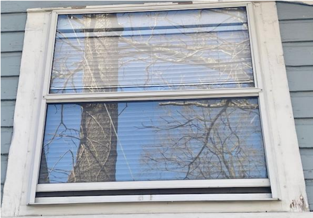
Existing window-east side
