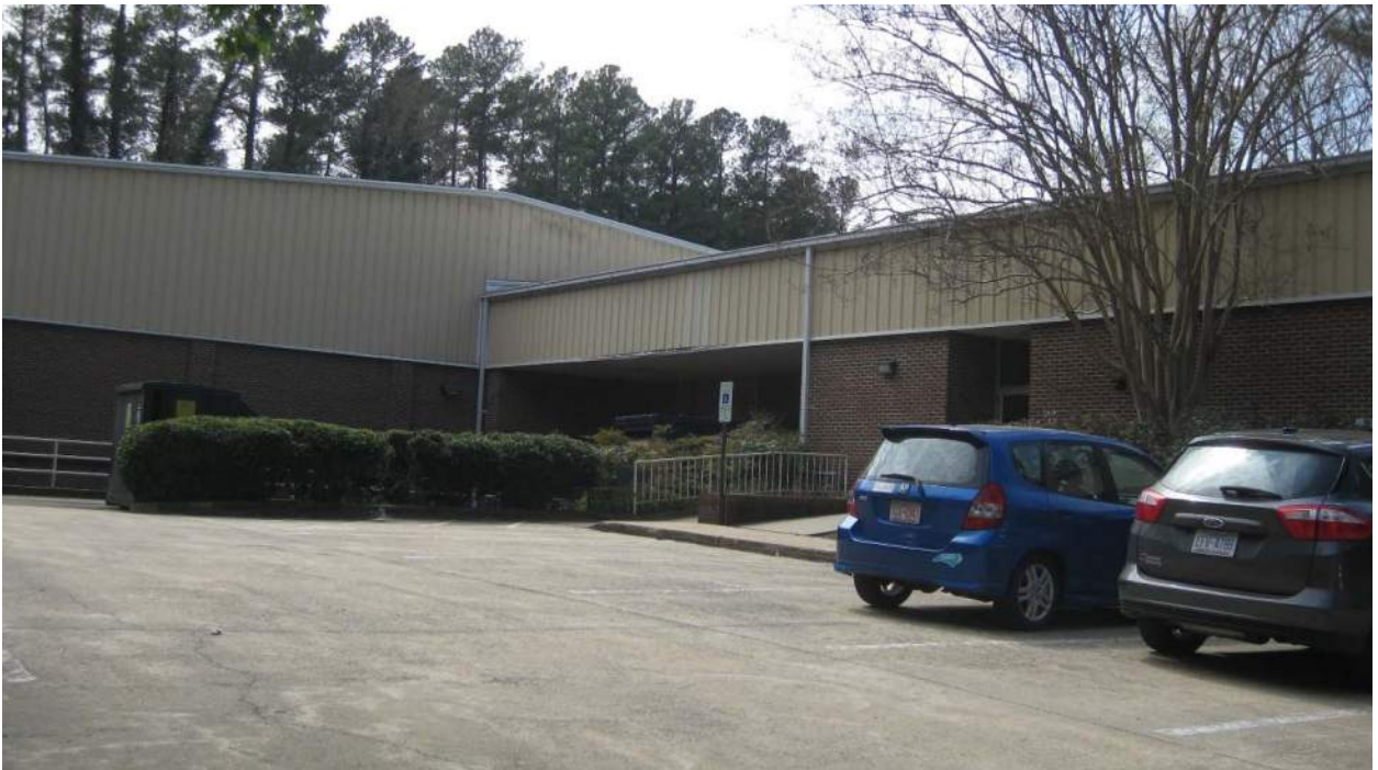
Municipal Buildings Contiguous to Justice Street
