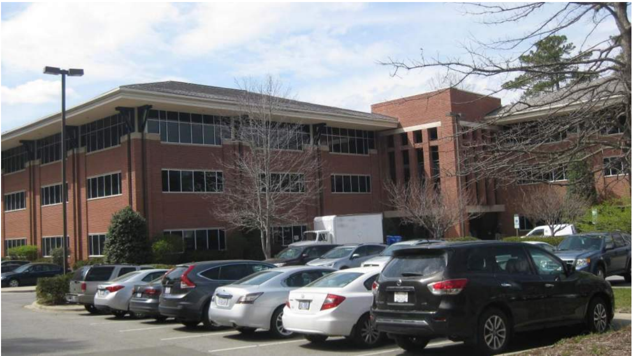
Municipal Building Contiguous to Justice Street
