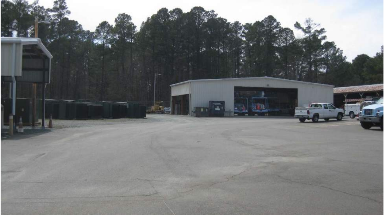
Municipal Building Contiguous to Justice Street
