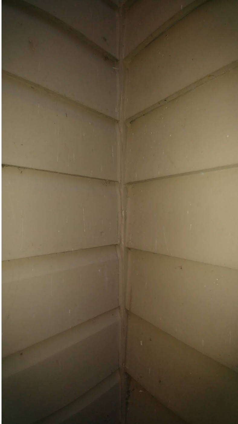
Allura Fiber Cement Lap siding (Right) compared to existing Masonite siding (Left)
