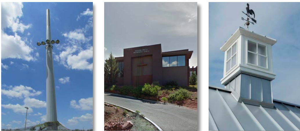
Figure 8: Concealed Base Stations - Light Stanchion - Building Concealment
