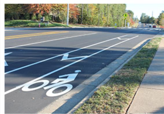
Public Facilities & improvements
