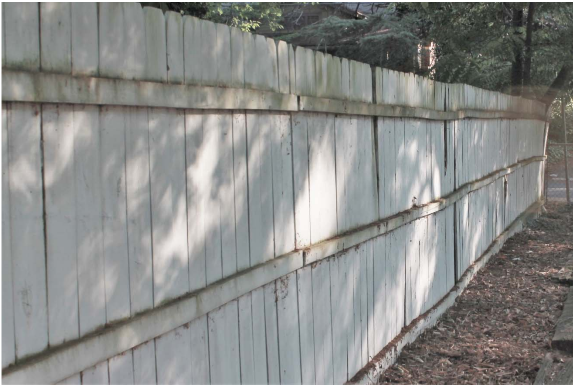
Kenan Street. On the boundary for the Historic District, this fence is used to screen parking from a residence. Although painted, the pickets are of the same dimensions and are dog-eared, but they do not alternate sides of the rails.
