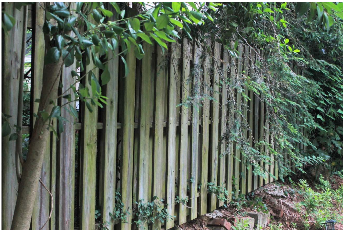
Existing picket fence. The proposed fence extends this fence line towards the middle of the block. This existing fence is almost identical to the proposed fence with the only difference being that the pickets on this fence are not dog-eared.
