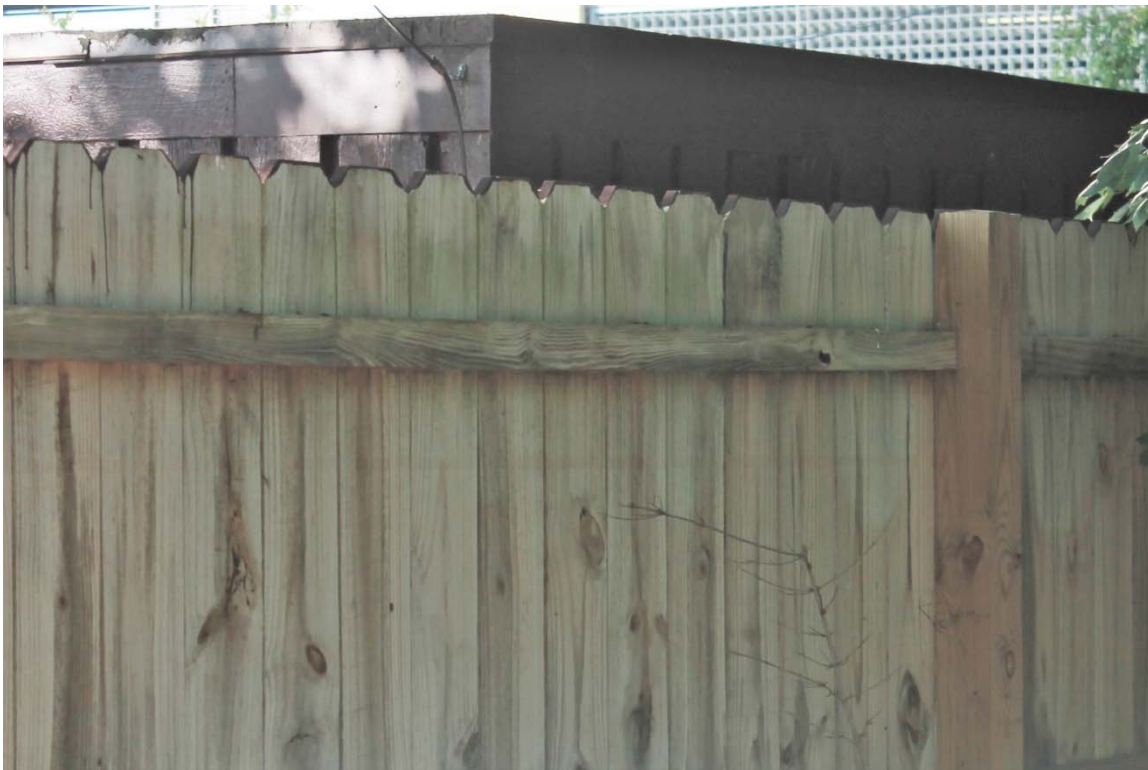
Mallette Street. Another fence used to screen a residence from parking. Identical or very similar materials although the pickets do not alternate sides of the rails.
