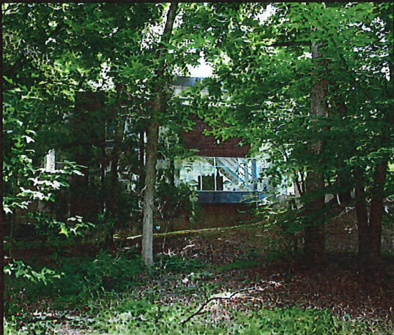
11. WEST ELEVATION VIEW FROM LOWER YARD.
