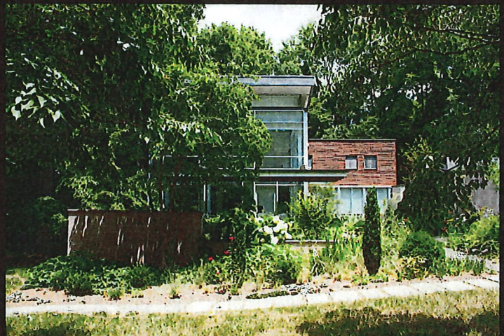
8. SOUTH ELEVATION VIEW, LOOKING NORTH FROM UPPER YARD TOWARDS MAIN ENTRANCE AND TERRACE.
