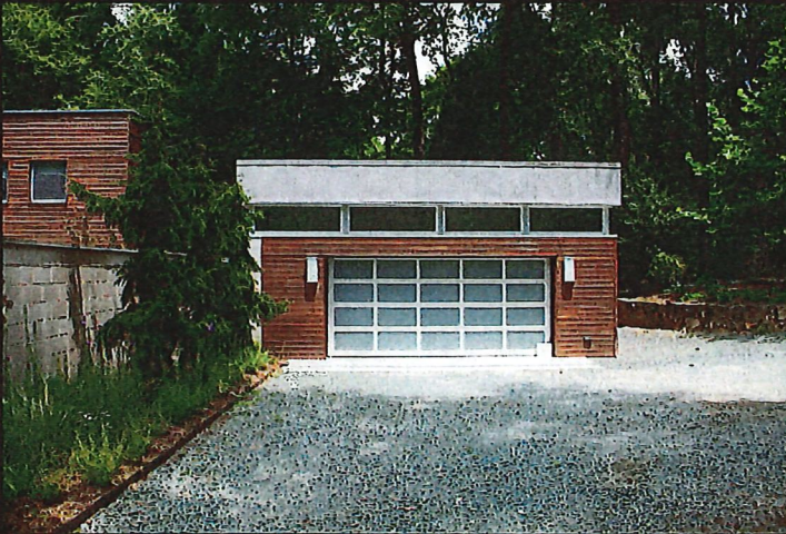
5. SOUTH ELEVATION VIEW OF GARAGE, LOOKING NORTH NEAR ENTRANCE GATE.
