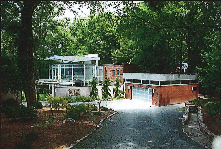
3. VIEW OF HOUSE NEAR THE END OF ENTRANCE DRIVE, LOOKING WEST.
