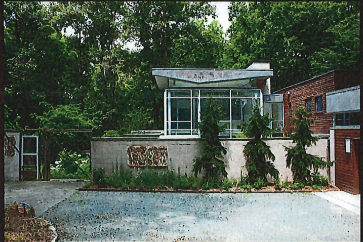
4. EAST ELEVATION VIEW, LOOKING WEST FROM DRIVE PARKING AREA JUST BEFORE THE GARAGE. MAIN ENTRANCE JUST BEYOND MASONRY WALL.
