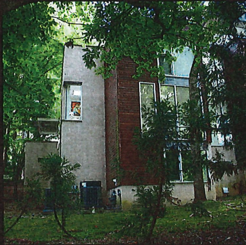
12. COMPOSITE WEST ELEVATION VIEW FROM LOWER YARD.
