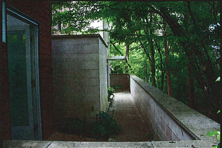
6. VIEW OF SIDE ENTRANCE WALKWAY FROM GARAGE, LOOKING WEST ALONG NORTHERN SETBACK.
