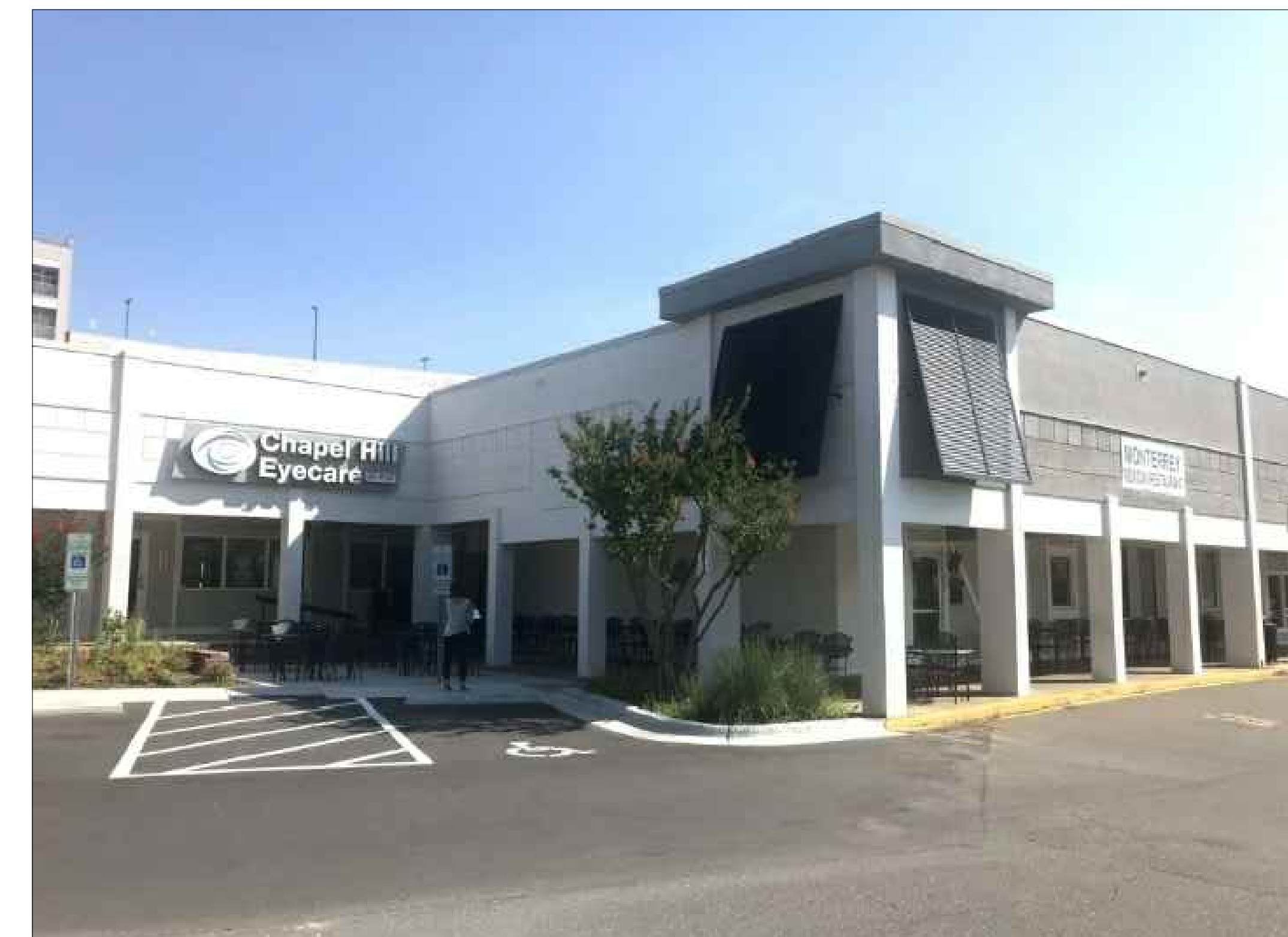
4 EXISTING- SUITES 235 + 237 - SOUTHWEST CORNER SCALE: NTS EC4
