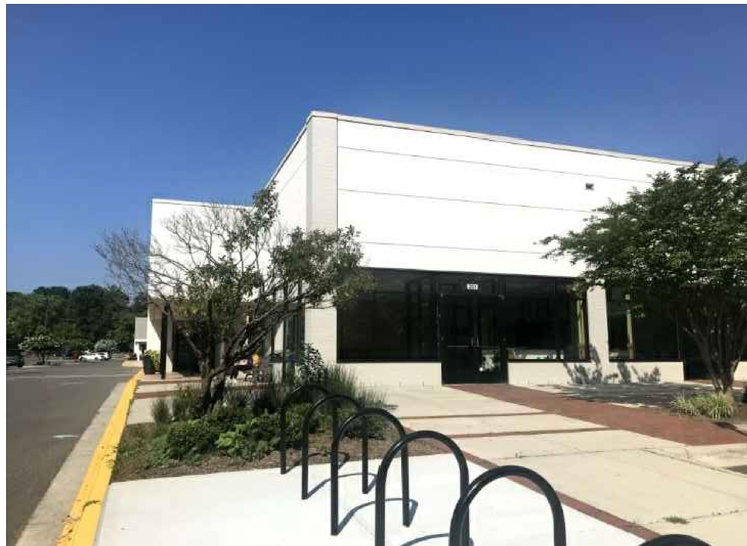
3 EC2 EXISTING- SUITE 261 - SOUTHEAST CORNER SCALE: NTS
