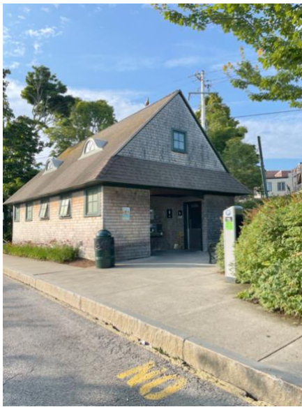
Figure 1 Public Restroom in Bar Harbor, Maine
