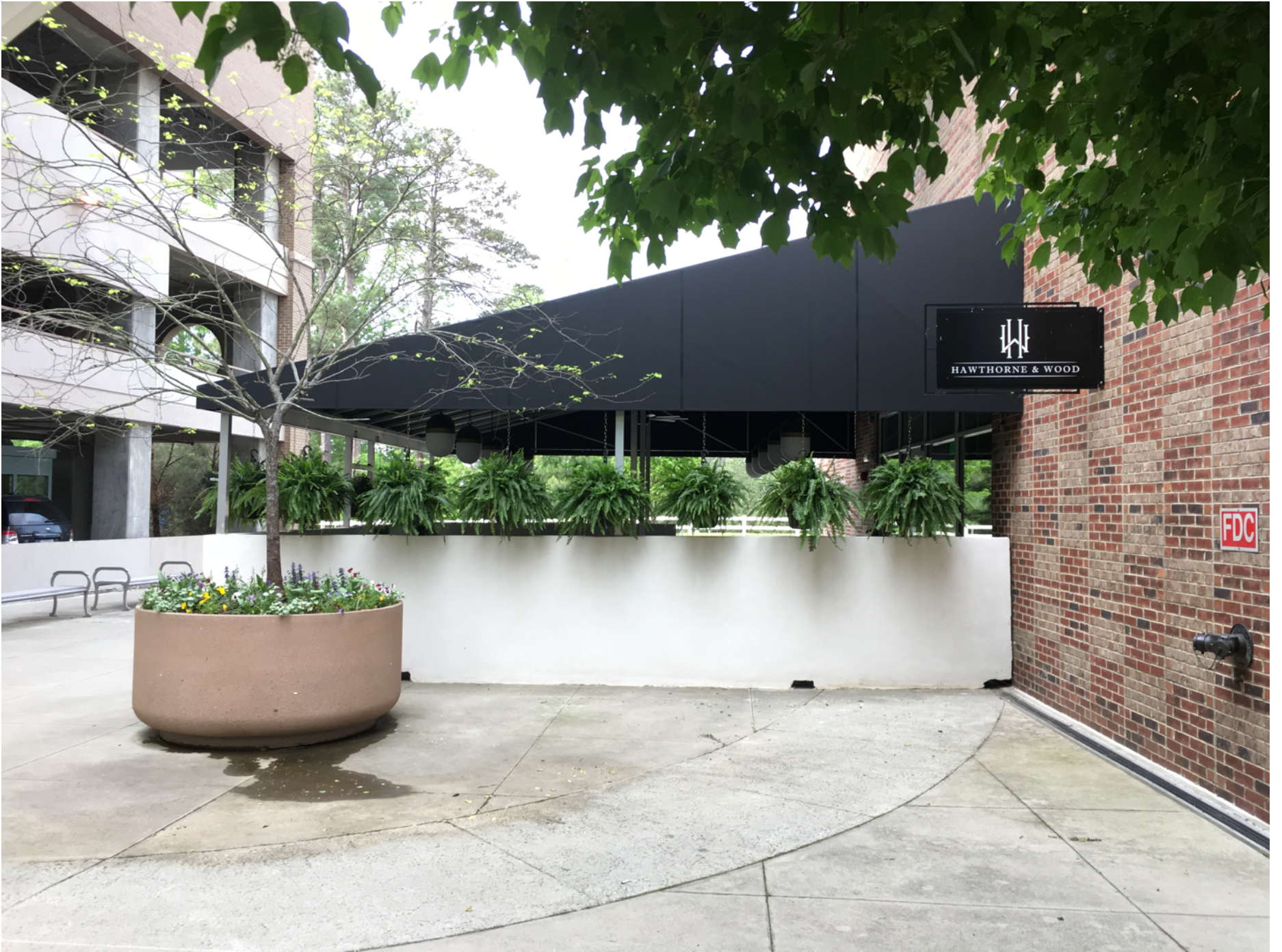
3. VIEW OF CANOPY AND PATIO FROM NORTH
