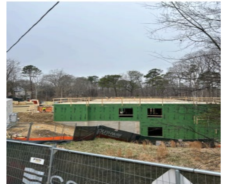
Public housing units demolished; new construction being erected
