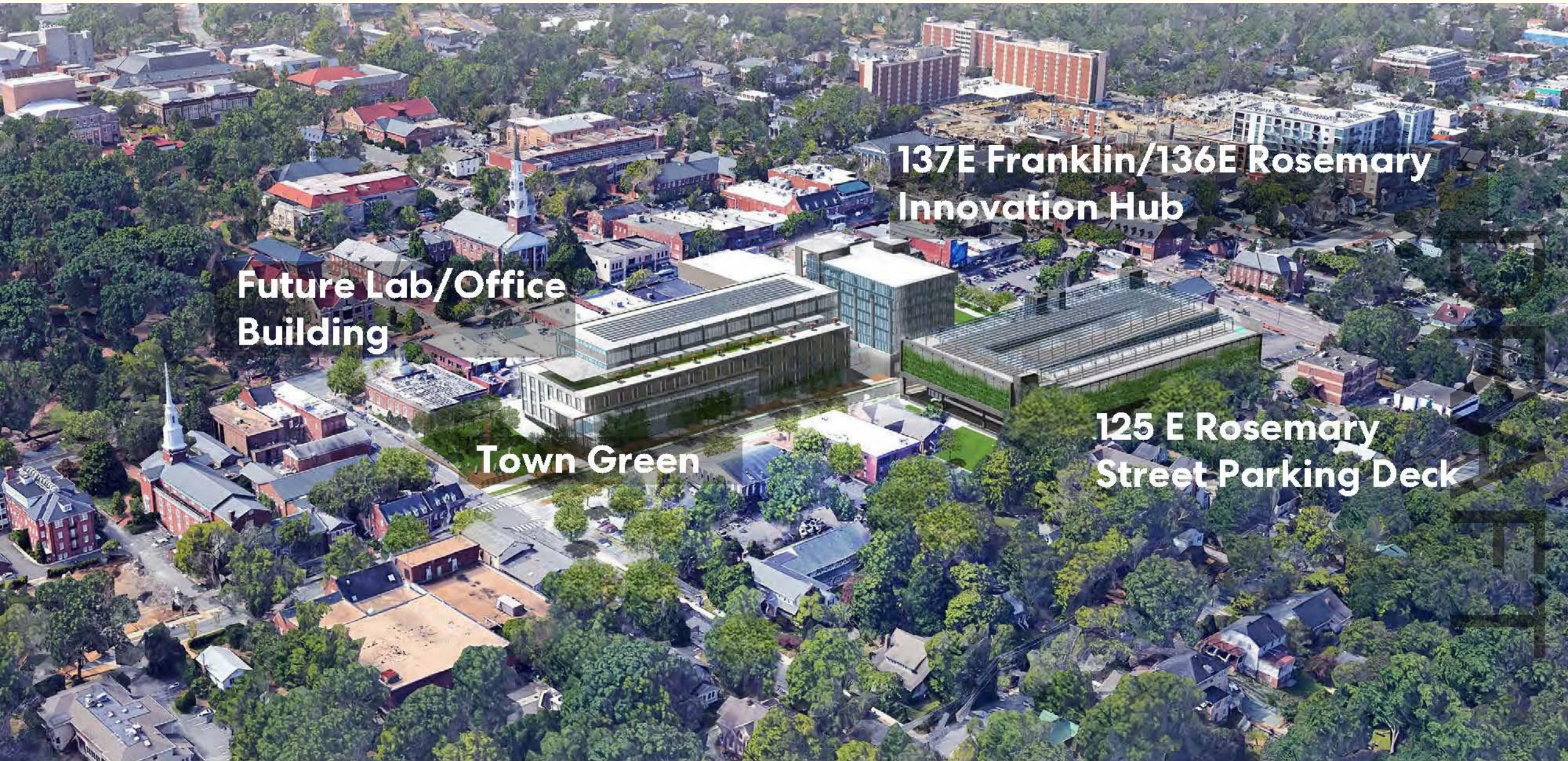
Aerial view from Northeast
