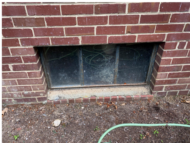
existing metal foundation vent/window
