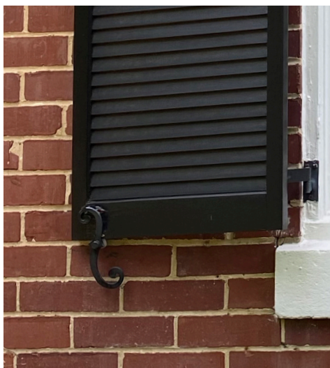
Existing shutter Detail- New shutter hinges & pintles and scroll shapes shutter dogs will match existing
