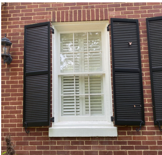
Existing Window Details to be replicated - 6 over 6 wood double hung window with operable shutters at primary facade
