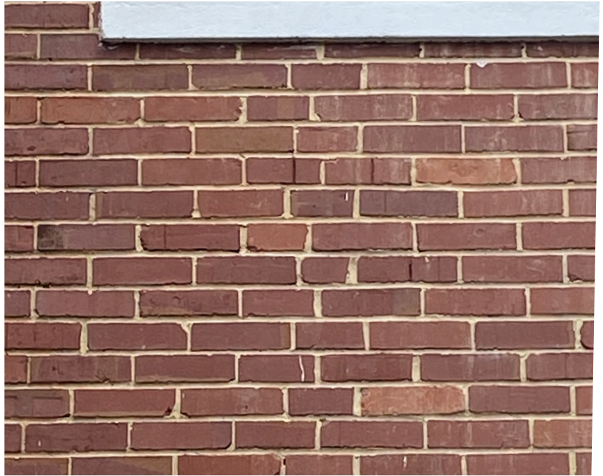
damaged, stained, and discolored brick and mortar at 214 Glenburnie
