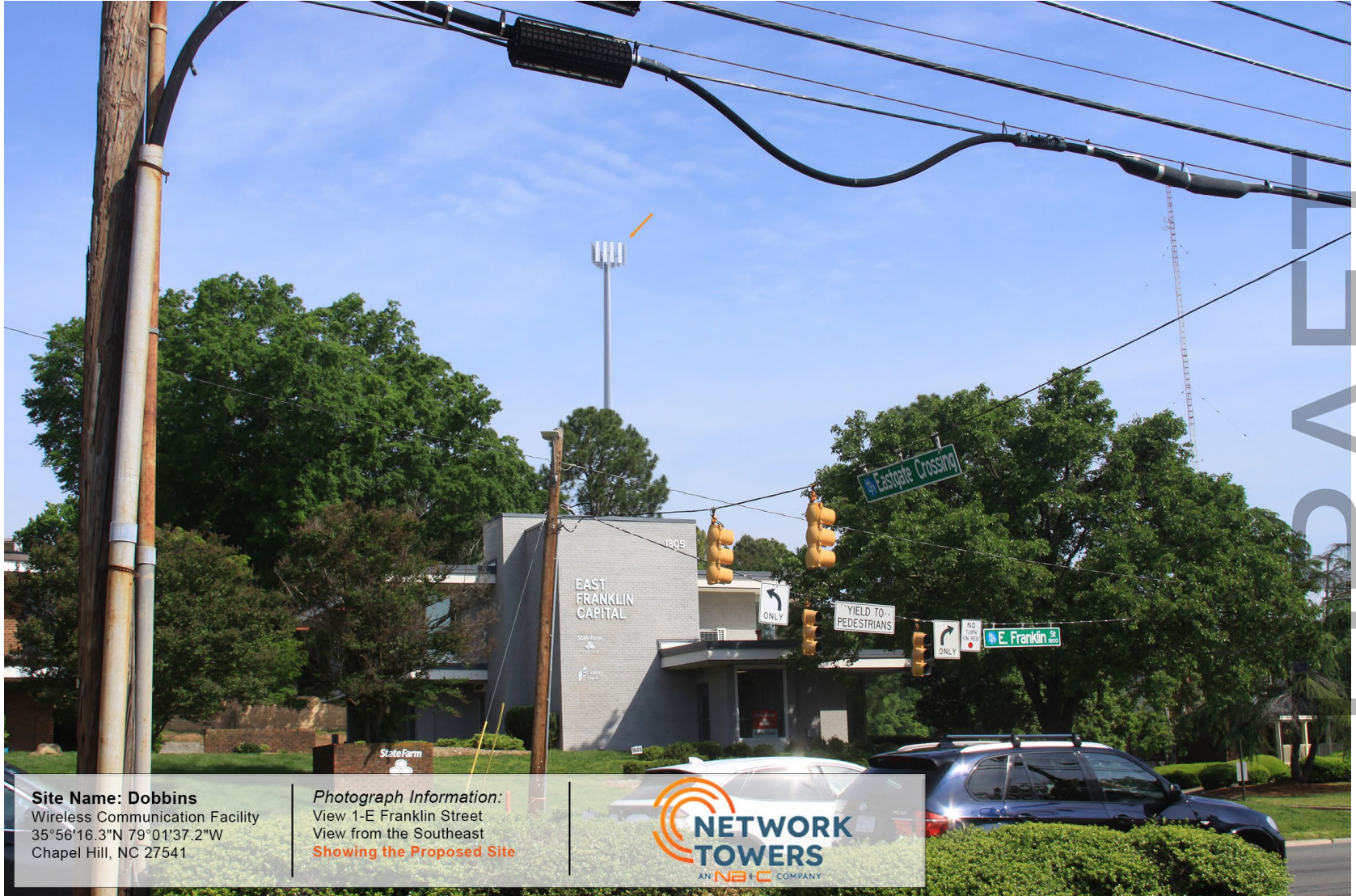
View 1 – E Franklin Street-View from the SE
