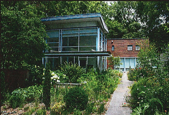
7. SOUTH ELEVATION VIEW, LOOKING NORTH FROM GARDEN TOWARDS MAIN ENTRANCE.
