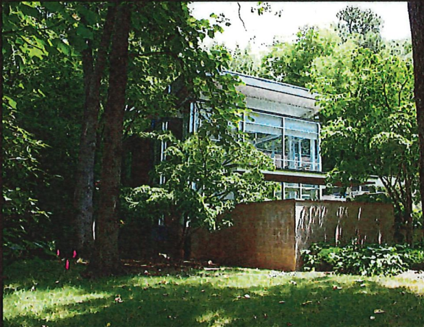
9. SOUTHWEST VIEW OF HOUSE, LOOKING NORTHEAST FROM MIDDLE YARD TERRACE.
