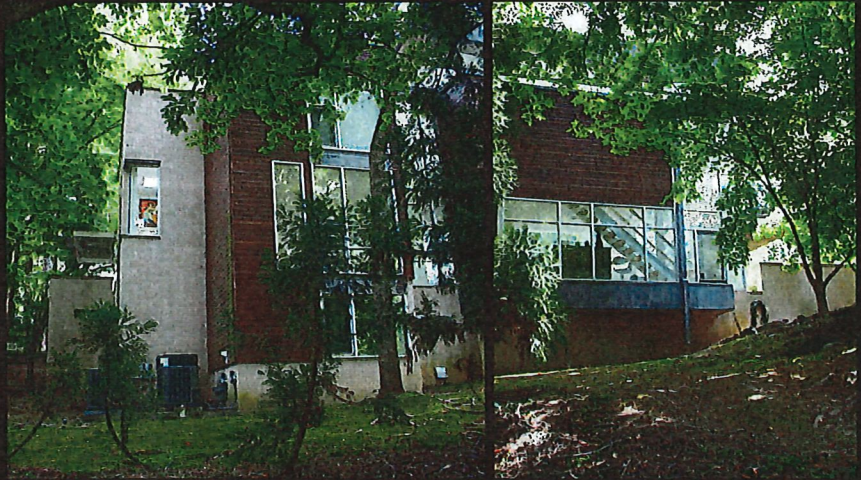
12. COMPOSITE WEST ELEVATION VIEW FROM LOWER YARD.
