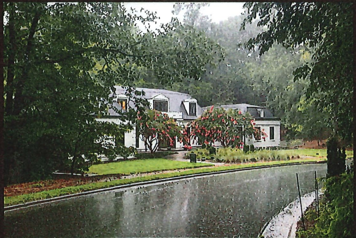
4. VIEW FROM 313 N. BOUNDARY STREET, LOOKING WEST TOWARDS 317 N. BOUNDARY STREET
