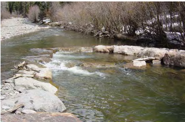
Figure 11-29 Cross vane structure with step on the East Fork Piedra River, CO
