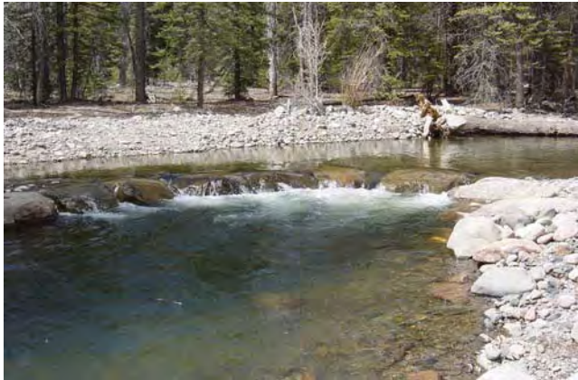
Figure 11-37 Native boulder J-hook with cut-off sill, East Fork Piedra River, CO
