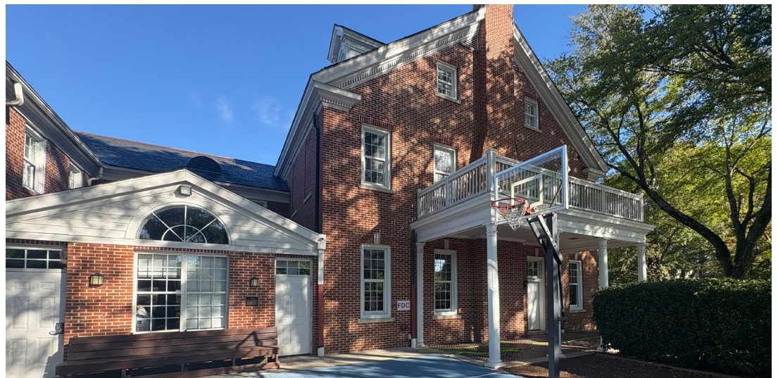
Area of Work
