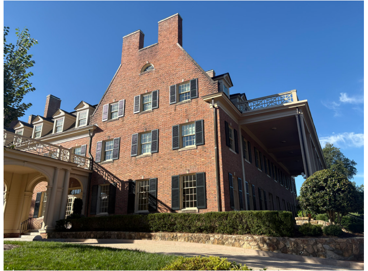
North East Corner
