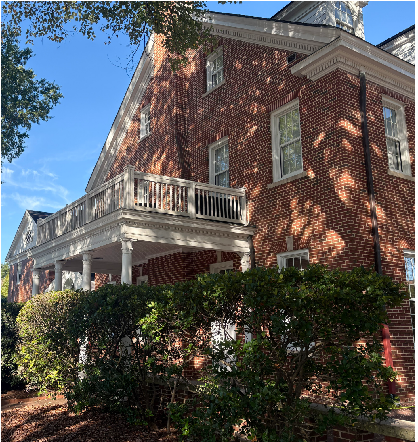
South East Corner
