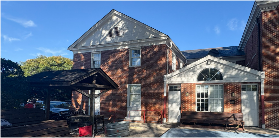
Area of Work
