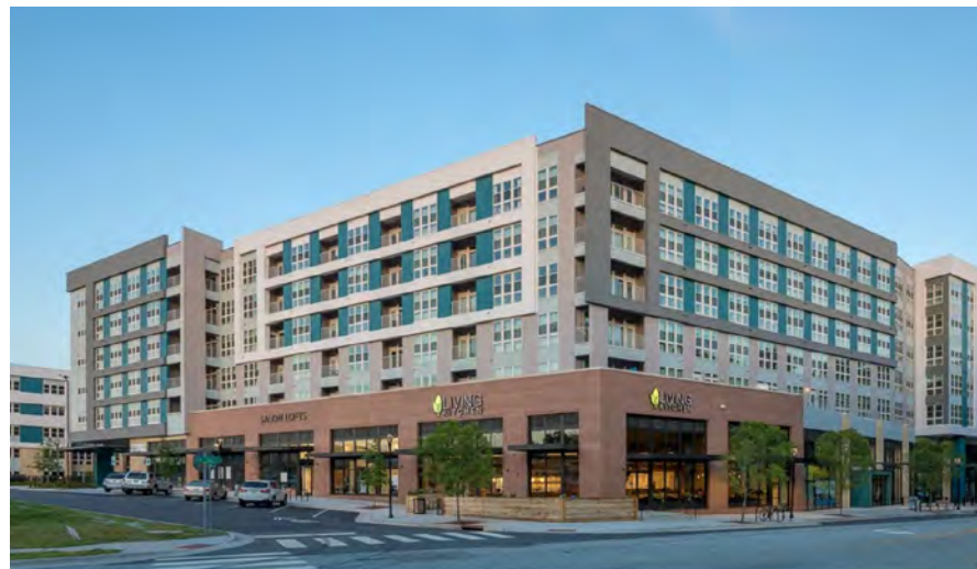
Berkshire Apartments from west
