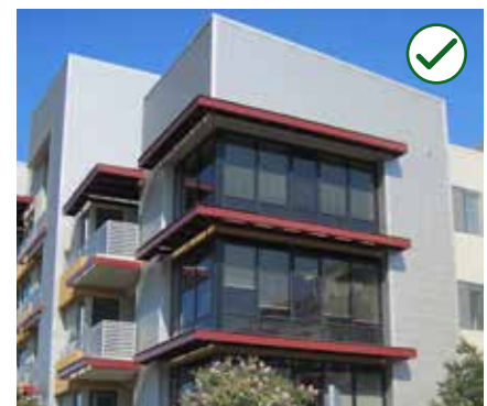
Figure 4-45 Architectural metal may be considered as a primary building material for design alternatives on building walls.
