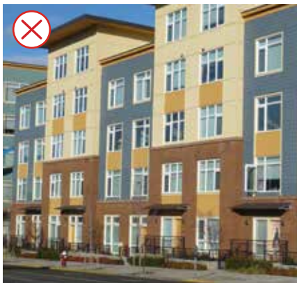
Figure 4-41a Avoid mixing several materials in a way that would result in an overly busy design.
