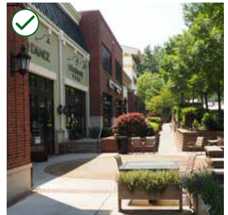
Figure 3-53c Consider locating a sloped sidewalk adjacent to stepped hardscape areas in order to maintain ADA access.
