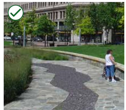
Figure 3-64 Incorporate Low Impact Development (LID) principles, such as stormwater planters and permeable pavement, to mitigate stormwater impacts.
