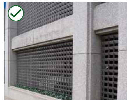
Figure 3-37 Design architectural screens to be an integral part of the building design.
