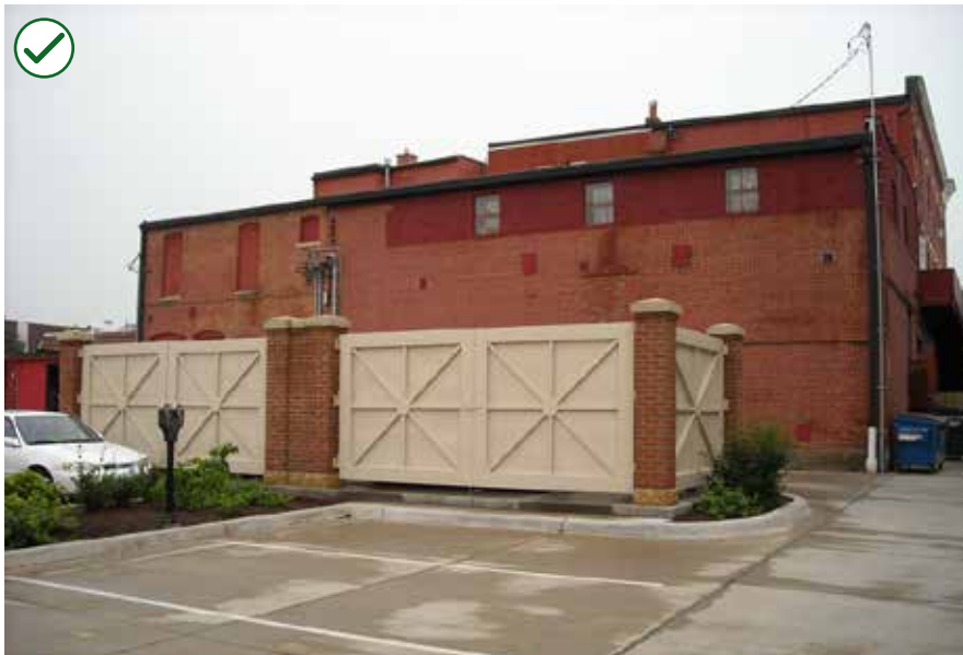
Figure 3-57b Use a similar material and color palette for service areas and utilities, when separate from a primary building.
