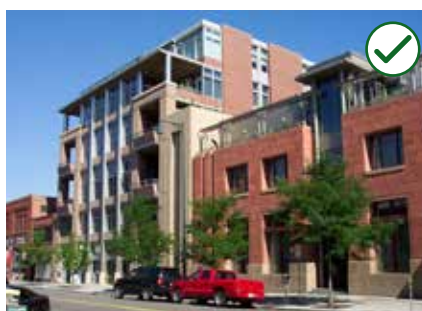
Figure 4-23b Use materials or other facade features that are compatible with adjacent buildings.
