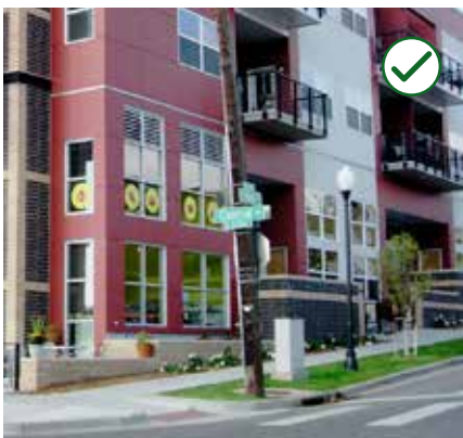
Figure 3-51 Design a building to step with the existing topography of a site.
