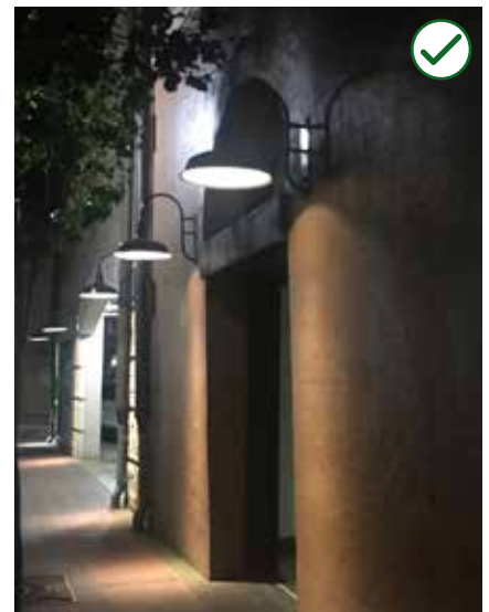
Figure 4-54 Use shielded and focused light sources to prevent glare and light pollution.
