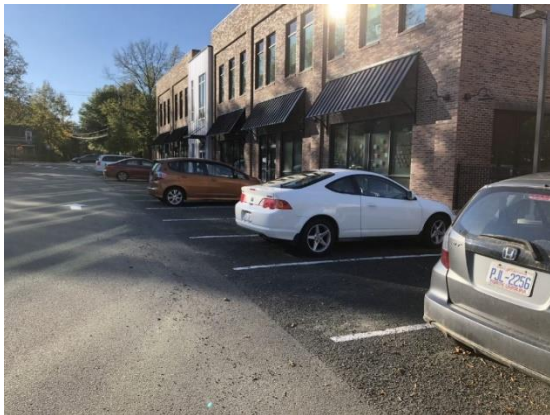
Pervious pavement in the parking space
