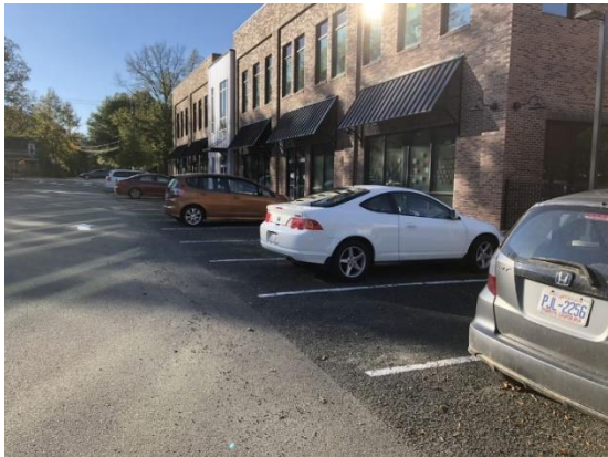
Pervious pavement in the parking space
