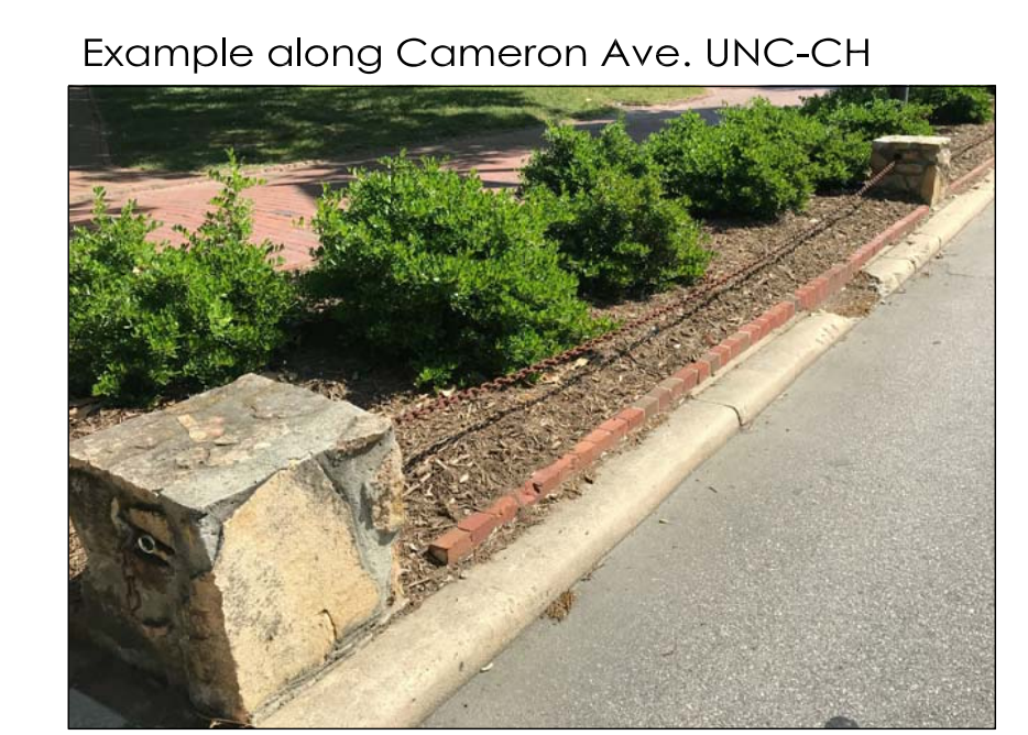
Example along Cameron Ave. UNC-CH Stone pier and chain
