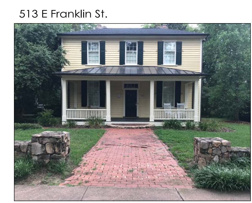
513 E Franklin St. Stone piers flanking walk
