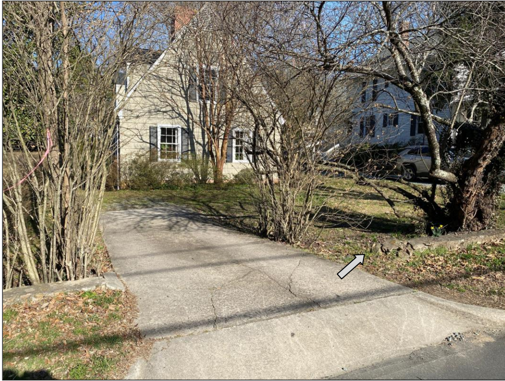
Views of existing concrete driveway and gravel parking area. A short section of the damaged rubble wall (arrow) will be removed to allow the new driveway to be 1 foot wider.
