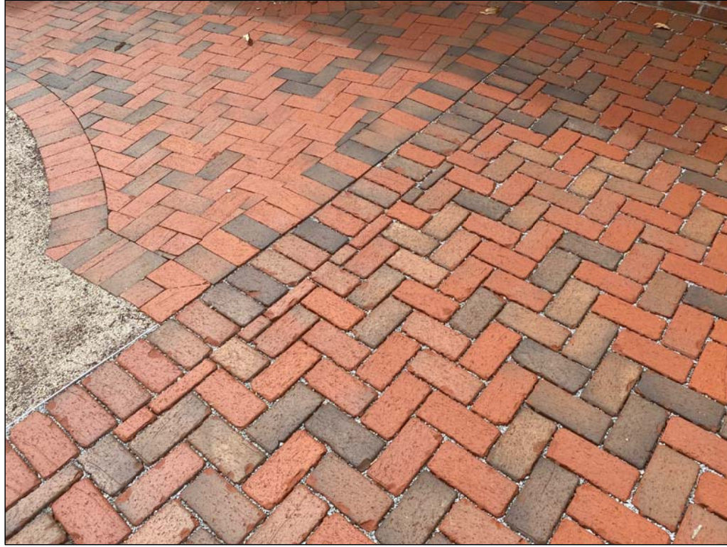
Driveway Storm Pave Permeable Pavers connection to front entry main walk using Pine Hall Pathway Full Range pavers
