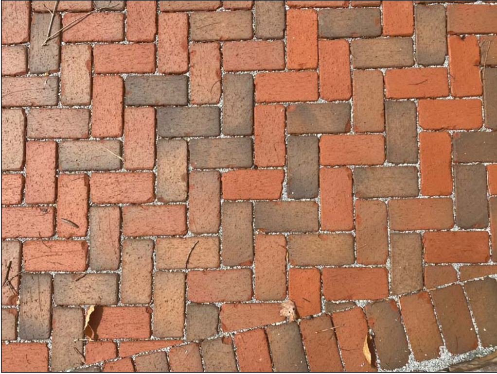
Pine Hall Rumblbed Full Range Storm Pave Detail Herringbone Pattern with 8" border
