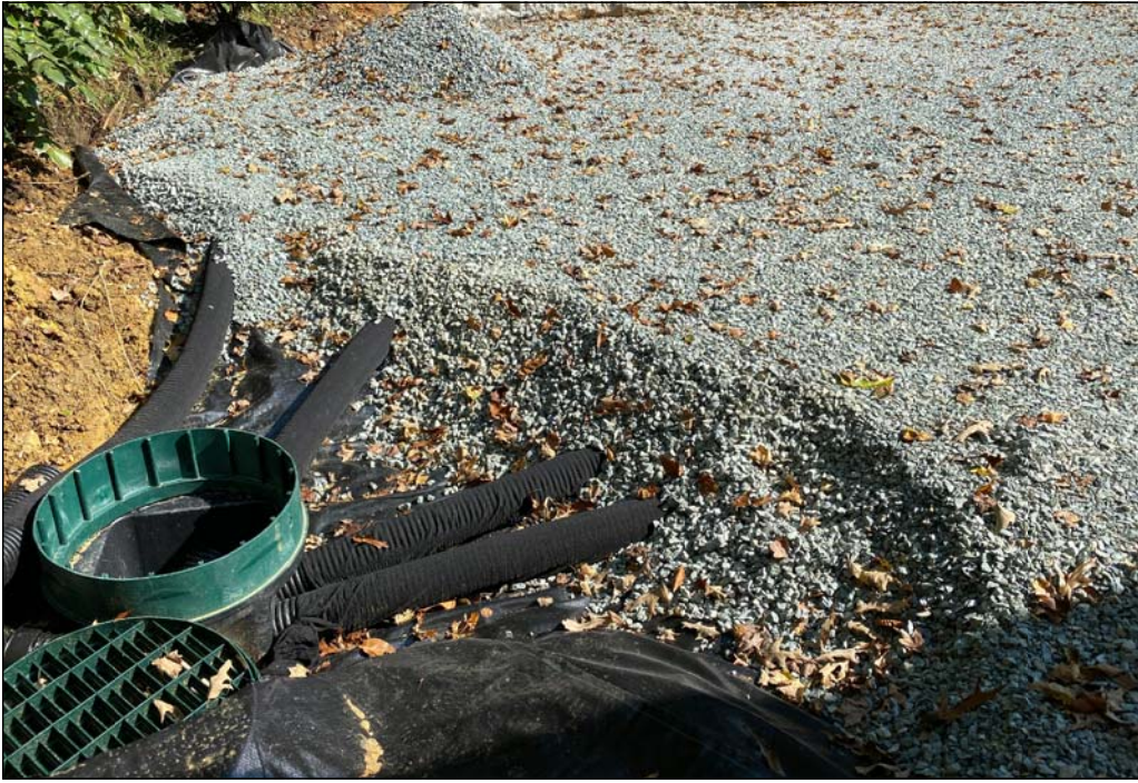
Sub-base gravel with filter cloth and undersdrains base for Storm Pave
