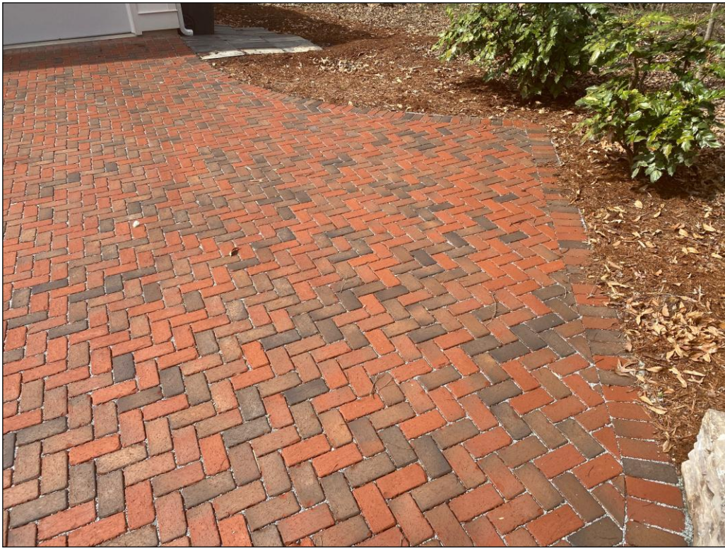
Example of the proposed driveway appearance, using Pine Hall Rumpled Full Range Storm Pave 2.25" brick pavers in a herringbone bond pattern. Instead of flat edging, matching bullnose brick edging will be used (refer to detail on plans.)
