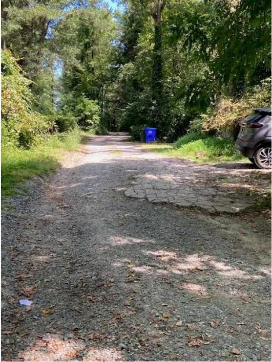
Looking north from south end of Huse Street road improvements
