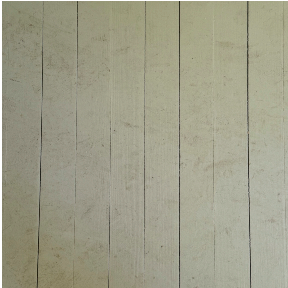
Pressure treated tongue and groove pine deck boards painted to match the existing wrap around porch/screened porch decking
