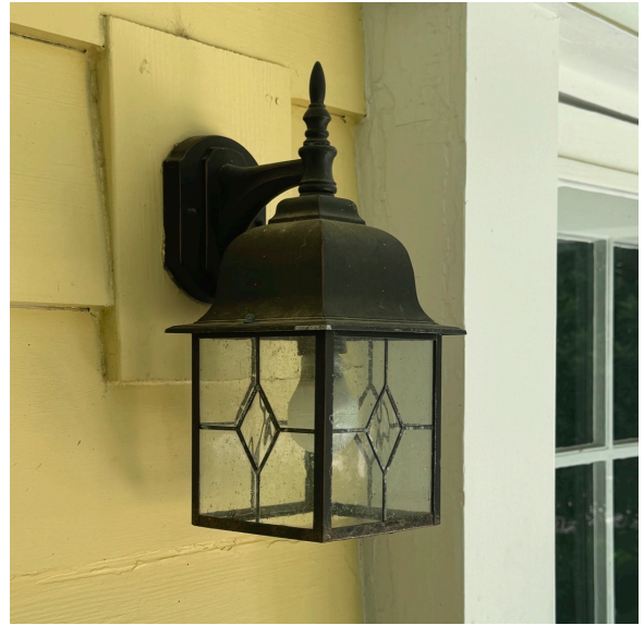
Existing wall sconce at entry
