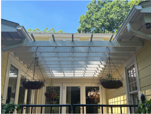
Existing non-original pergola at existing rear southern addition
