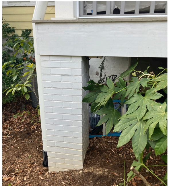
Existing non-original brick pier at wrap around porch/screened porch
