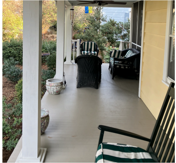
Existing deck at wrap around porch
