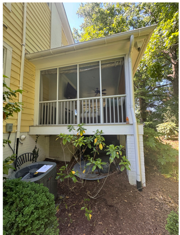
side (east) screened porch - location of proposed deck addition
