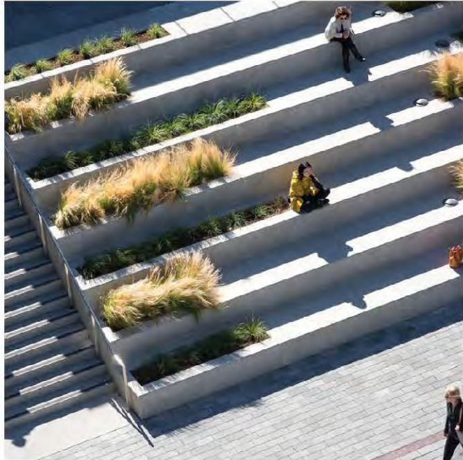
LIMESTONE COLOR PRECAST WALLS & STEPS
