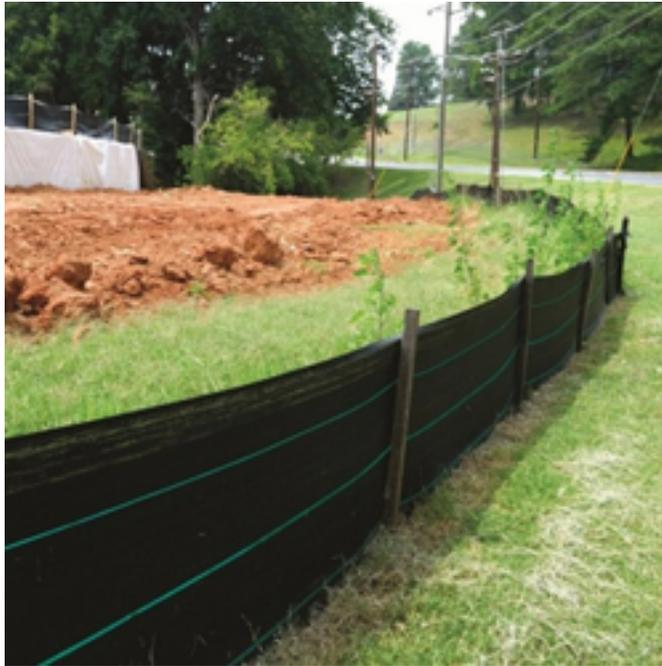
Photograph 1: Standard silt fencing
