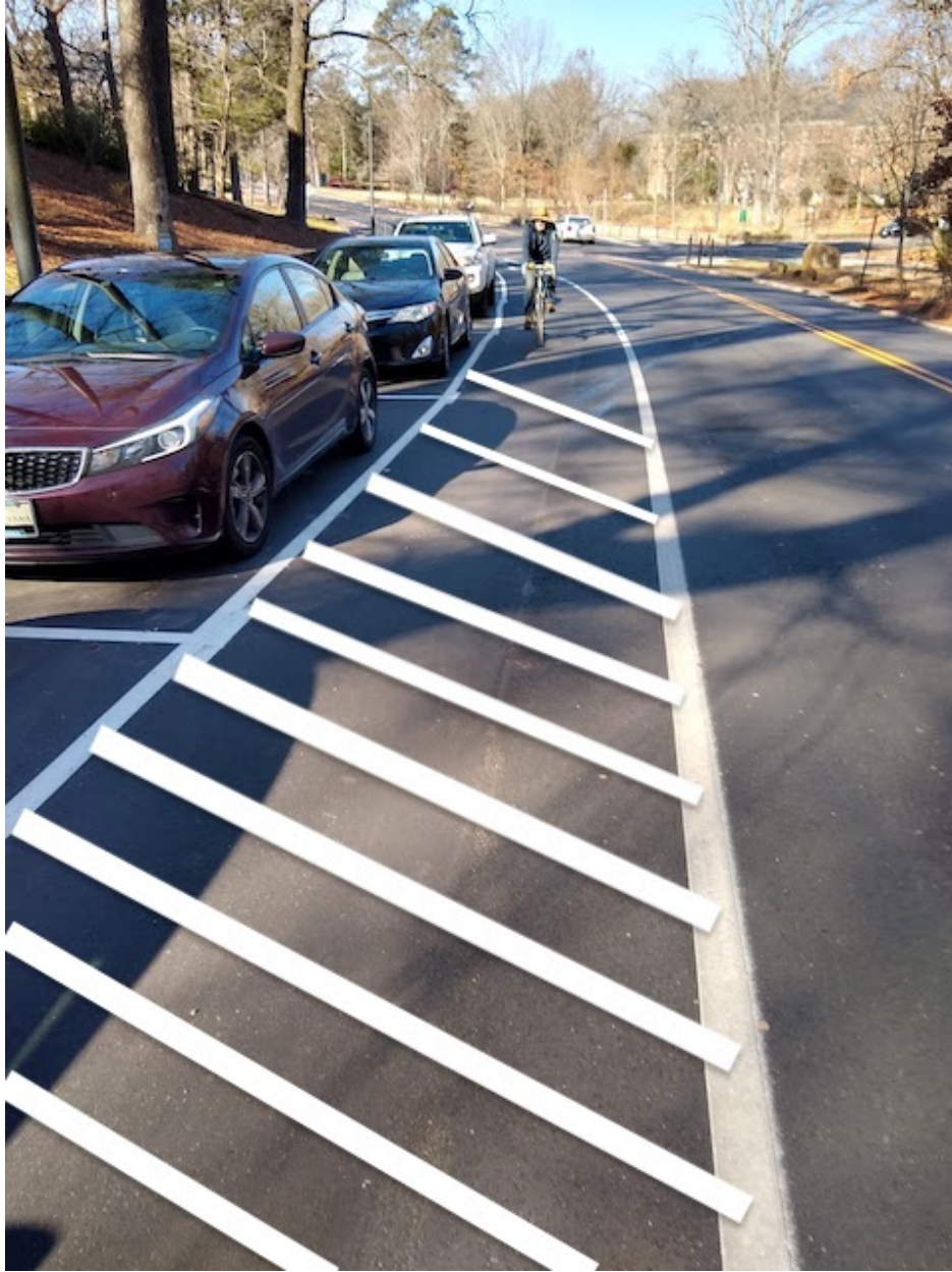
Image 3. Rather than a Bike Lane, it should be a buffer showing the area to avoid.
