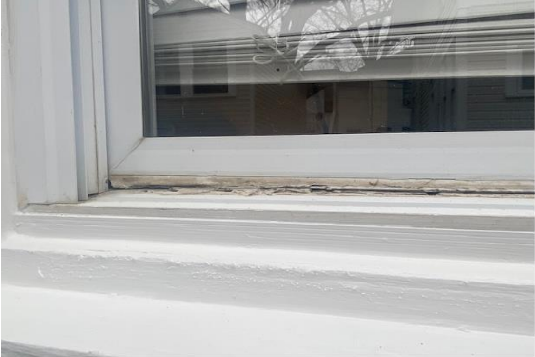
View of existing window-west rear side
