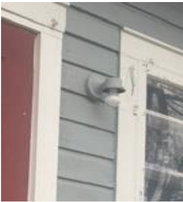
Existing side porch light
