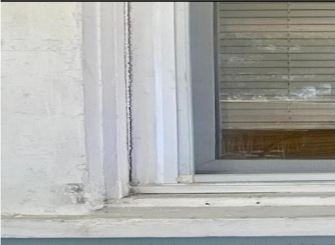
Closer view of existing vinyl windows-front of house
