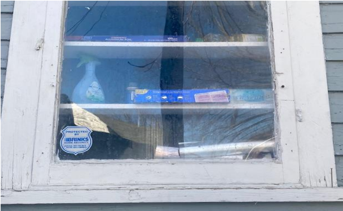
Existing window-east side (near side porch)-this one is not vinyl-perhaps original
