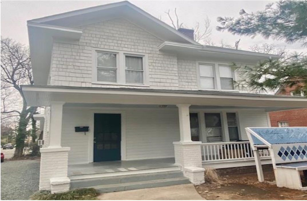
View of front of house-south side
