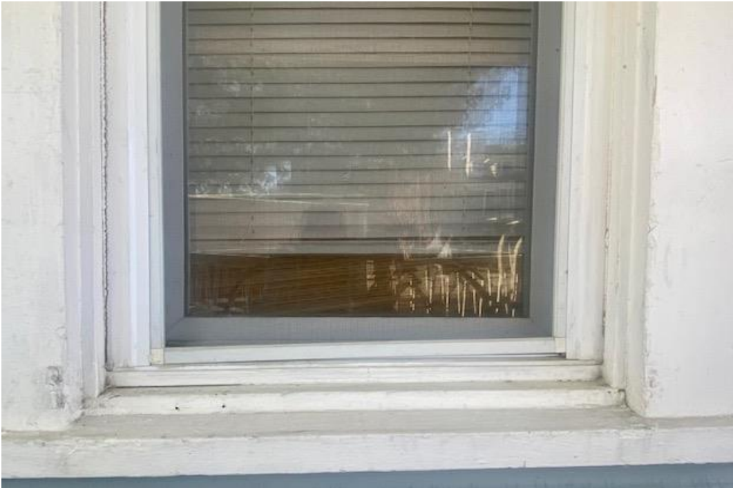
Closer view of existing vinyl window-front of house
