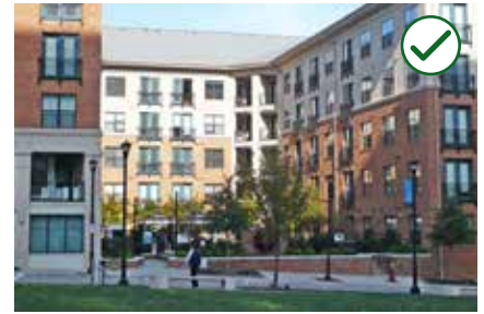
Figure 4-35 Expanding the width of a forecourt may be considered as a design alternative when the edge is clearly defined.
