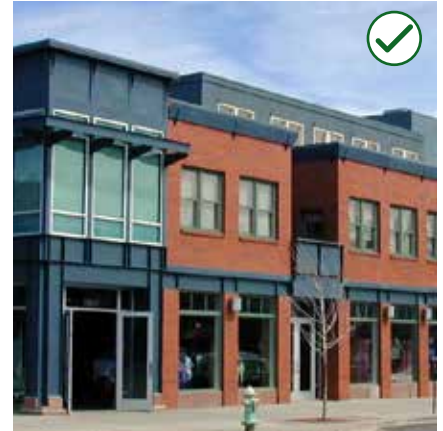
Figure 4-26 Use building materials to define the ground floor and add visual interest.
