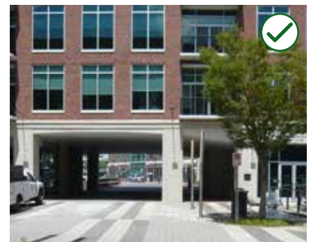
Figure 3-11 Design a building pass-through to be inviting and in proportion to its associated building.
