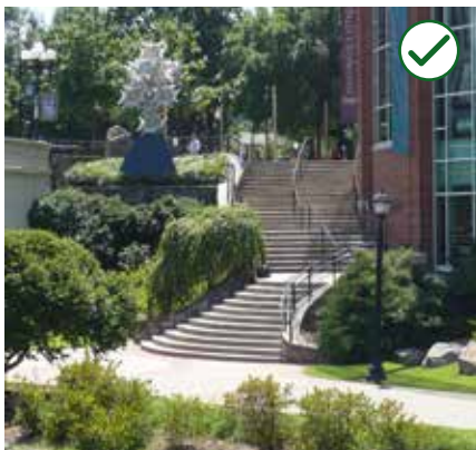
Figure 3-48b Use a series of landscaped terraces or stepped walls where a taller cut or change in grade is necessary.
