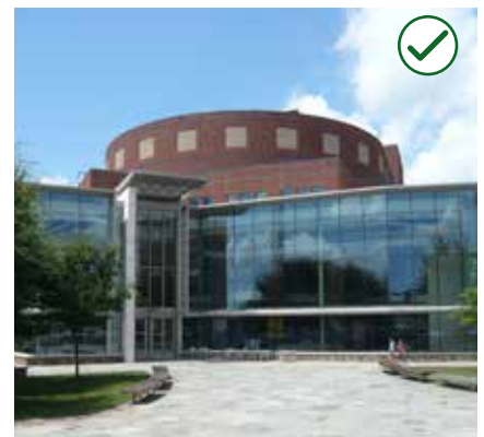
Figure 4-28 Orient the primary entrance of a building to face a street, plaza or pedestrian way.
