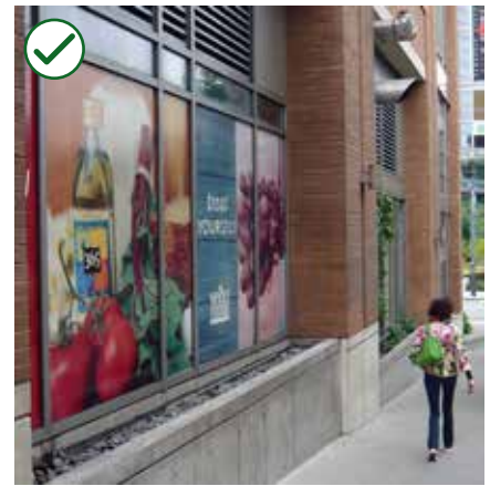
Figure 3-52 Integrate the elements of a building facade to respond to changes in topography.
