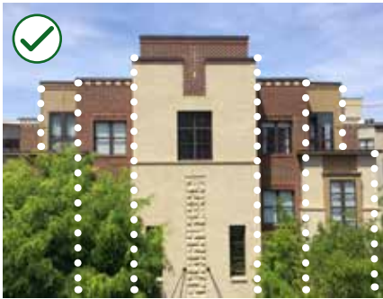
Figure 4-15 Provide vertical articulation in a larger building mass to establish a sense of scale.
