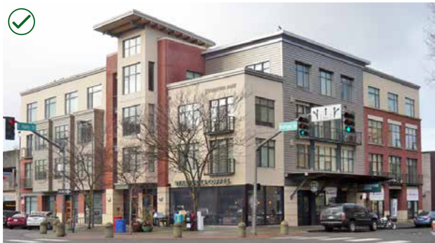
Figure 4-31 Locate an iconic design feature to maximize its visibility and impact. For instance, locate the feature at the primary building entry,
