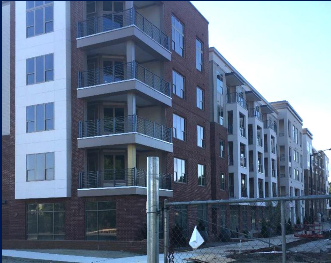
Frontage along Novus Ln Looking west towards Fordham Blvd
