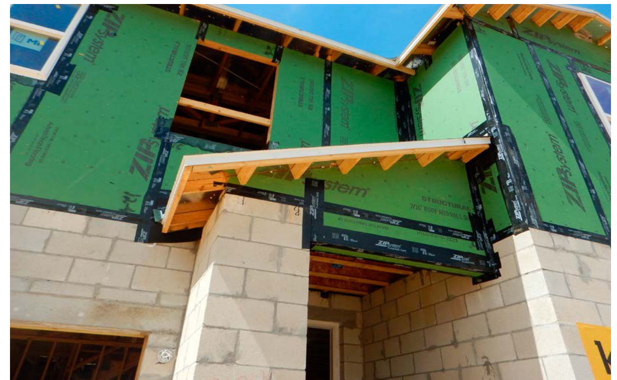
KB home under construction in Orlando, Fla.
