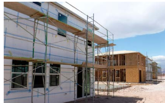
Scaffolding at a KB Home community
