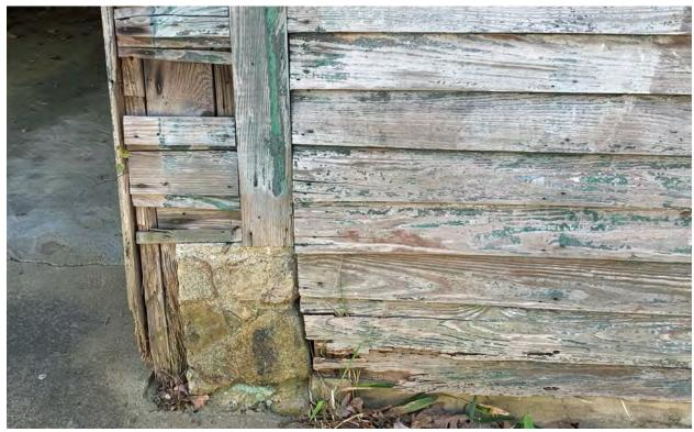
Water and termite damage is evident throughout the exterior wall framing and sheathing.
