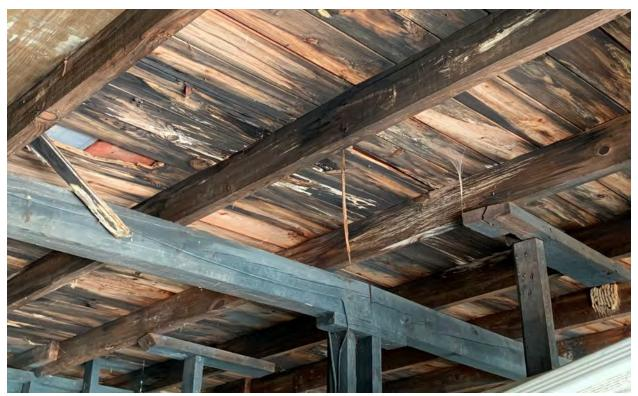
The existing garage was constructed in multiple phases on top of a mix of stone and brick foundations, resulting in differential settlement. The above photo shows some of the differential settlement at the north wall + typical fascia damage due to failure of the existing metal roof.
