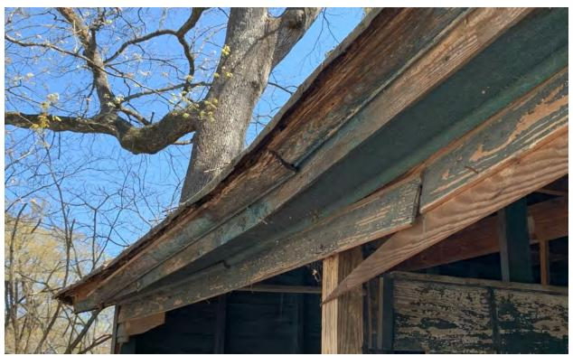
Failure of the standing seam metal roof has resulted in extensive water damage to roof framing, sheathing, and fascia.
