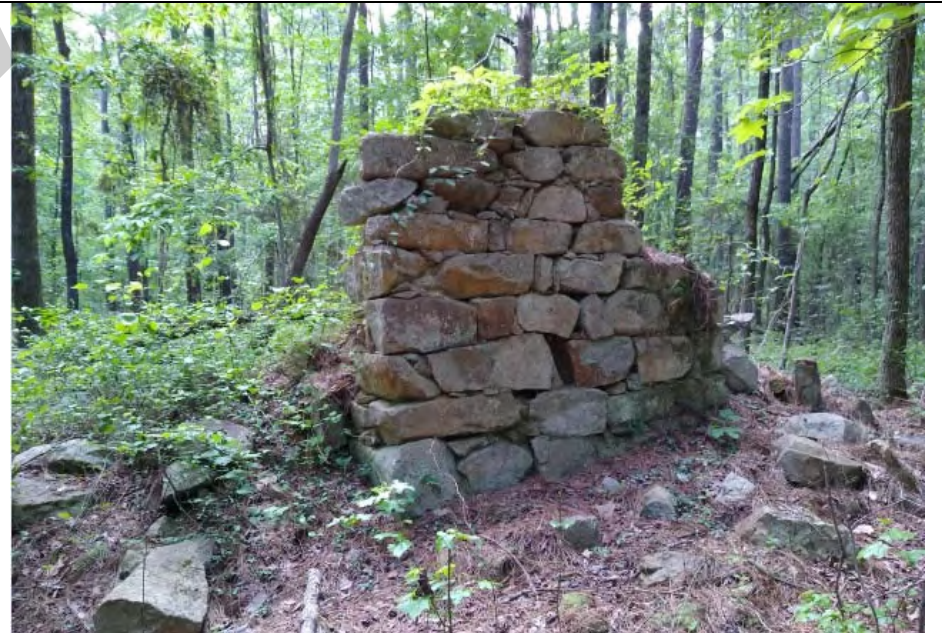
Potts homestead chimney remains, near Bolin Cr Reach C2/D1
