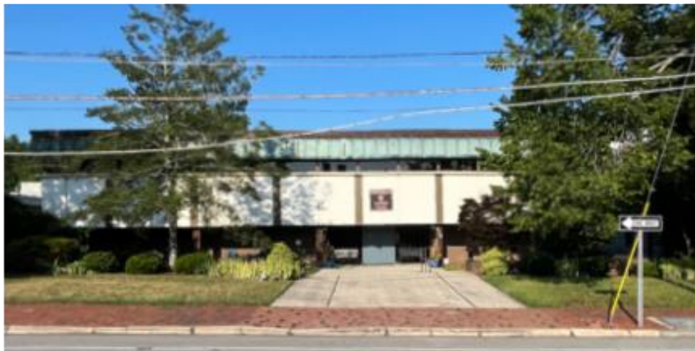
Street Facing Elevation. Materials: copper mansard roofing, framed ribbon window, precast concrete panels with reveals at joints, metal panels between concrete panels, concrete columns, brick, brick pavers.
