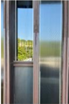
Mix of obscure and clear glass, frame reveal and flat faces, and recessed glazing units
