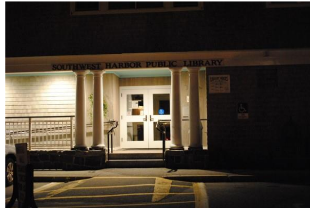
A light source where the bulb is not visible, and the light is directed downward. The light creates a safe environment for walking up to the building.
