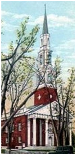
University Methodist Church Bell Tower 1926
