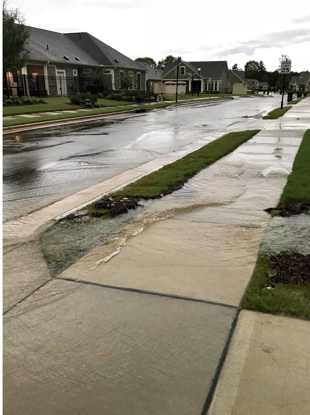
Flooding on the sidewalk in front of Lot 17
