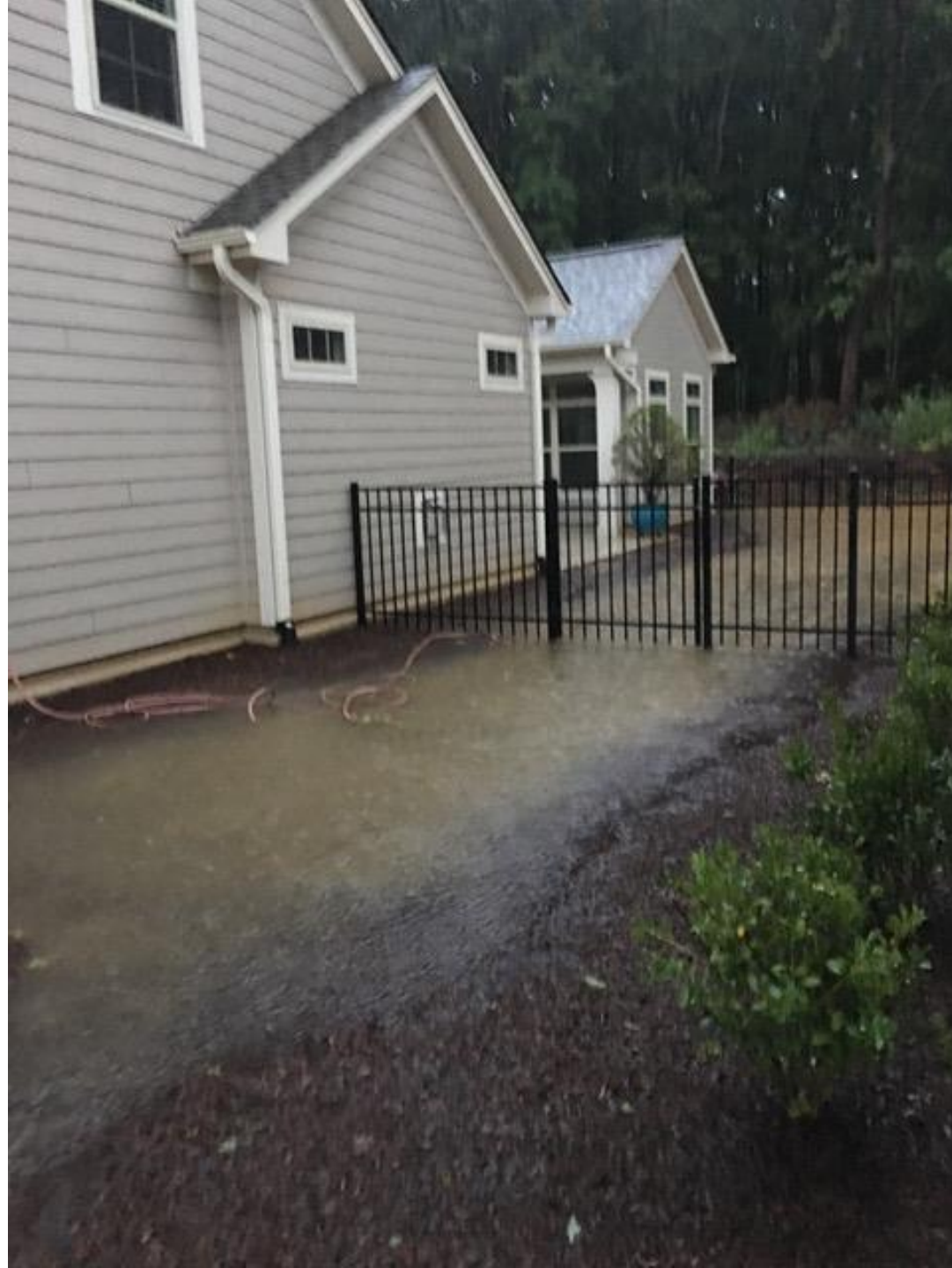
Flooding between Lots 13 and 14
