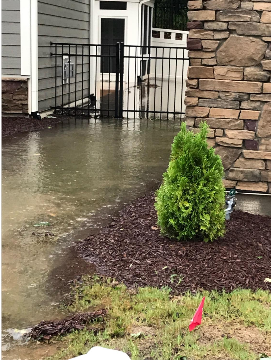
Flooding alongside Lot 17
