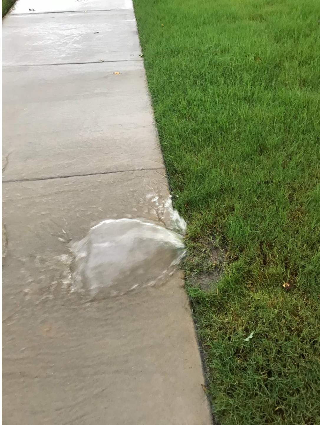
In ground pop-ups overwhelmed by flooding
