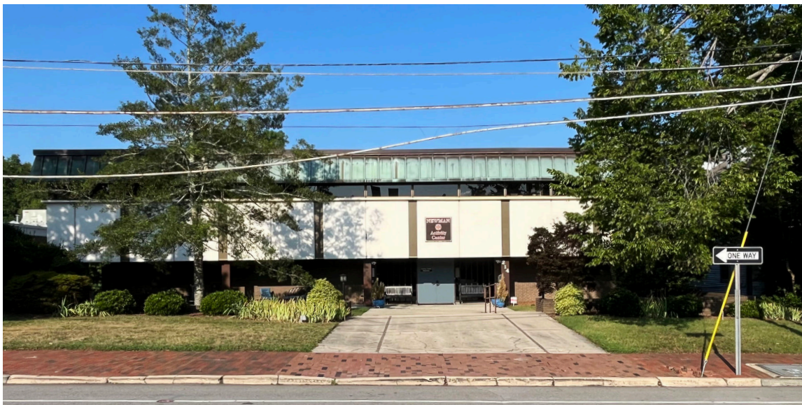
Street Facing Elevation. Materials: copper mansard roofing, framed ribbon window, precast concrete panels with reveals at joints, metal panels between concrete panels, concrete columns, brick, brick pavers.
